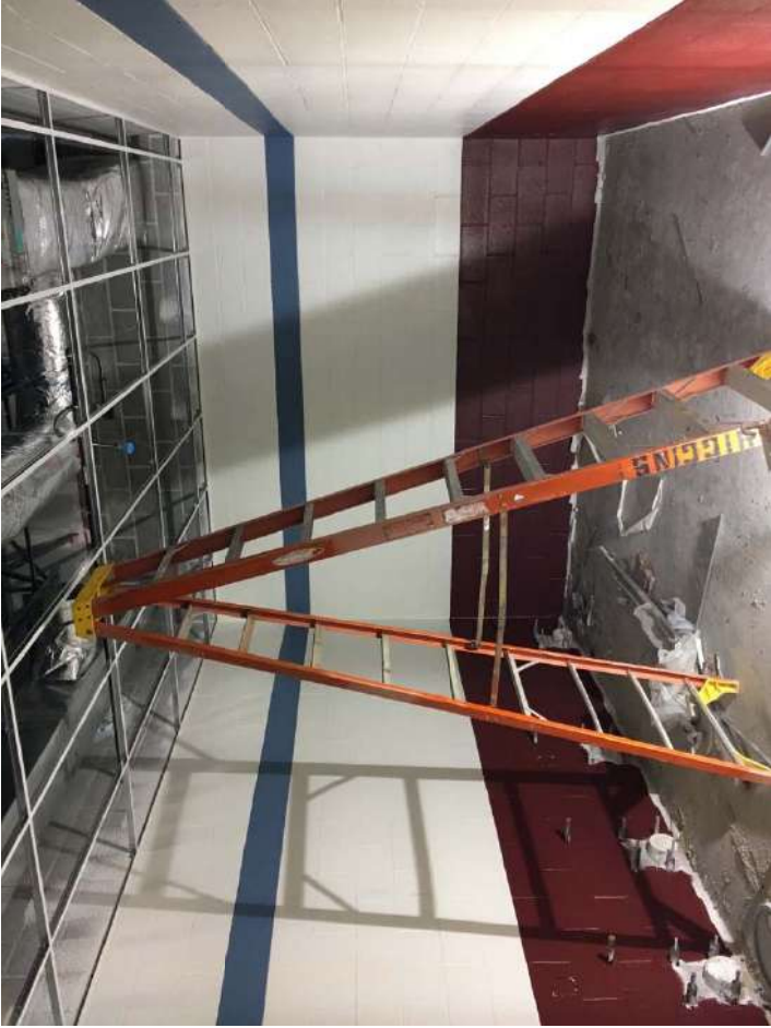
PAINTING UNDERWAY IN THE SOUTH CLASSROOM WING RESTROOMS.
