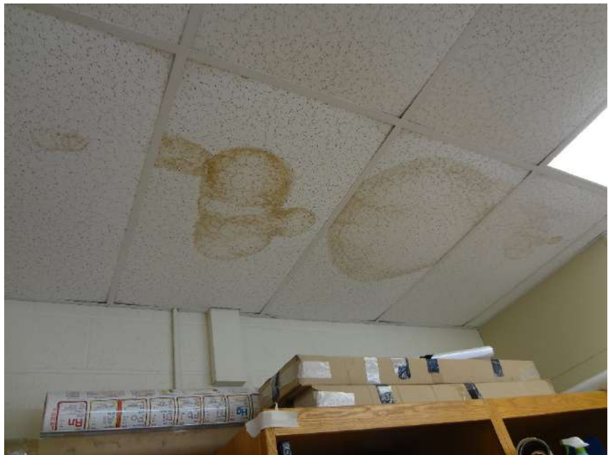
25. WATER STAINED CEILING TILES INDICATE A POTENTIAL OF WATER INFILTRATION AT ROOF - INVESTIGATE SOURCE OF MOISTURE AND REPAIR. REPLACE CEILING TILES
