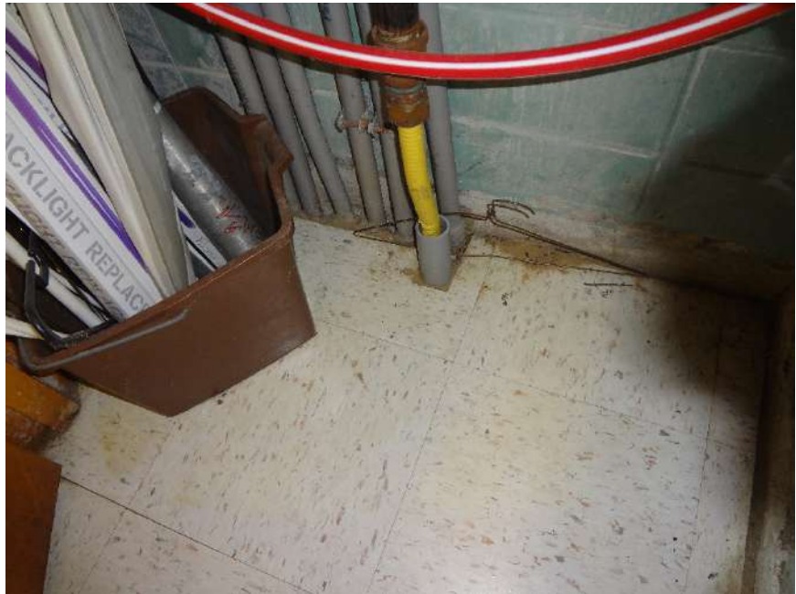
24. AREA OF WATER AND SAND INFILTRATION INTO CLASSROOM DURING HEAVY RAINS - CAMERA (INSPECT) UNDERGROUND STORM LINE TO DETERMINE CAUSE, REPAIR
