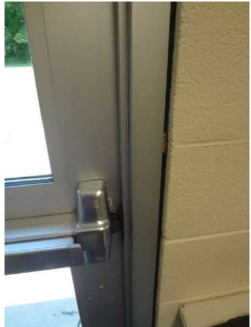
40. ENLARGED IMAGE OF MISSING BACKER ROD + SEALANT AROUND DOOR FRAME - INSTALL BACKER ROD AND CAULK AROUND FRAME, INSPECT WEATHERSTRIPPING
