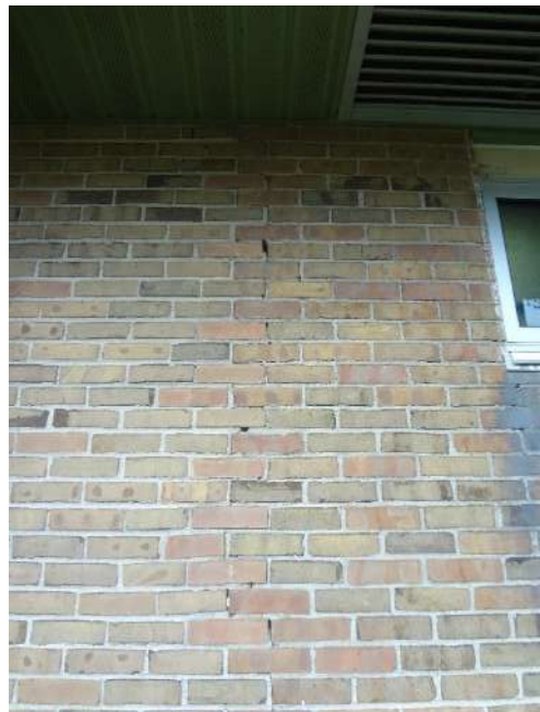
6. BROKEN + MISSING BRICK + ERODED GROUT THROUGHOUT AREA OF FAÇADE - CLEAN & REPOINT MASONRY AS NEEDED FOR DAMAGED JOINTS. INSPECT ANNUALLY.
