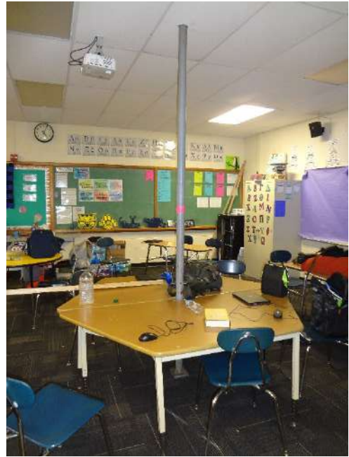
28. RETROFIT STEEL JACKPOST AT CENTER OF CLASSROOM - CONSULT STRUCTURAL ENGINEER TO MONITOR AND DETERMINE REPAIR SOLUTION
