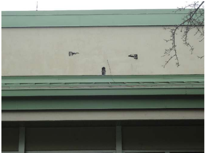
10. PUNCTURES IN EIFS, ALLOWING AIR + WATER INFILTRATION INTO ROOF CAVITY - PATCH AND REPAIR EIFS, FINISH TO MATCH EXISTING
