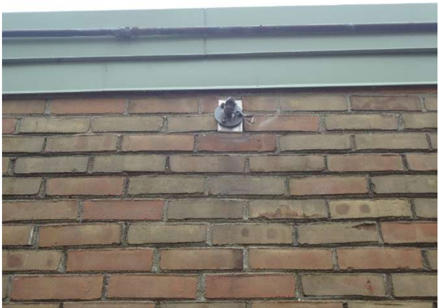
34. BROKEN EXTERIOR LIGHT FIXTURE ARM + MISSING EXTERIOR LIGHT FIXTURE - REPLACE EXTERIOR LIGHT FIXTURE
