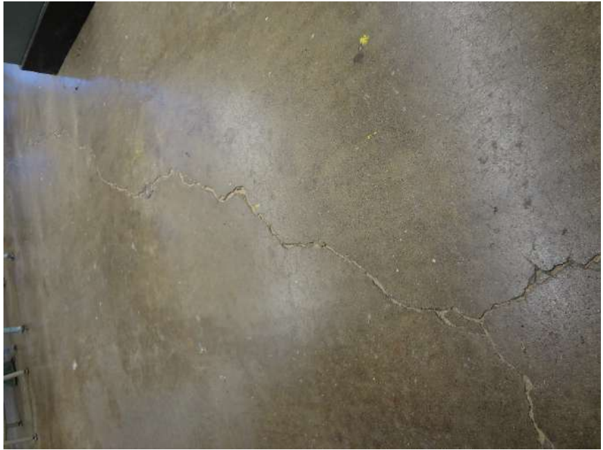
26. CRACKING IN CONCRETE FLOOR THROUGHOUT SHOP AREA - CRACKING IS INHERENT IN CONCRETE. MONITOR FOR MOVEMENT, FINISH IF DESIRED
