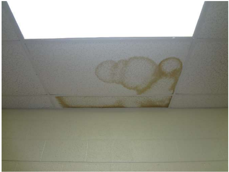
30. WATER STAINED CEILING TILES INDICATE A POTENTIAL OF WATER INFILTRATION AT ROOF - INVESTIGATE SOURCE OF MOISTURE AND REPAIR. REPLACE CEILING TILES
