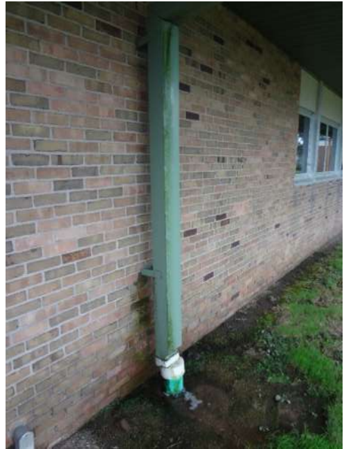
15. WATER LEAKING FROM TOP OF DOWNSPOUT, ORGANIC GROWTH ON FACE - CLEAN, INSPECT AND REPAIR DOWNSPOUT CONNECTION AS REQUIRED
