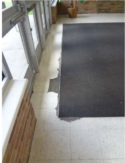
18. BROKEN VCT AT VESTIBULE ENTRY FROM WATER INFILTRATING UNDER DOORS, TYPICAL - STOP WATER INFILTRATION. FLOOR REPLACEMENT IN 2019, PART OF SINKNG FUND PROJECT
