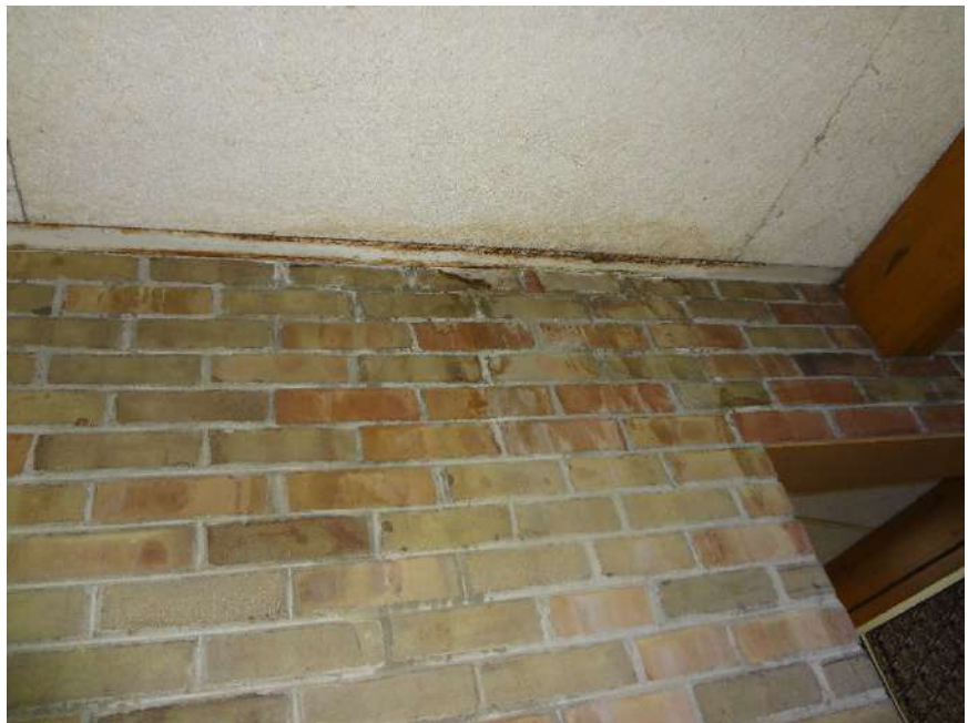
38. CORROSION OF METAL FRAMING, STAINING FROM MOISTURE INFILTRATION - INVESTIGATE SOURCE OF MOISTURE AND REPAIR. CLEAN BRICK AND CEILING ASSEMBLY
