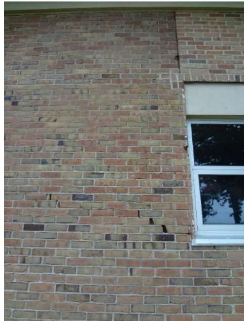
5. BROKEN + MISSING BRICK THROUGHOUT AREA OF FAÇADE - CLEAN & REPOINT MASONRY AS NEEDED. INSPECT ANNUALLY.
