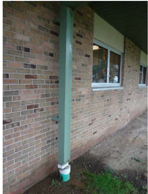
16. ANOTHER DOWNSPOUT LEAKING FROM SEAM AT TOP OF DOWNSPOUT - CLEAN, INSPECT AND REPAIR DOWNSPOUT CONNECTION AS REQUIRED
