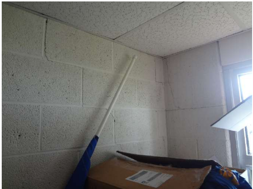
21. MASONRY CRACKS THROUGHOUT SOUTHEAST CORNER OF STORAGE ROOM - CONSULT STRUCTURAL ENGINEER TO MONITOR AND DETERMINE REPAIR SOLUTION
