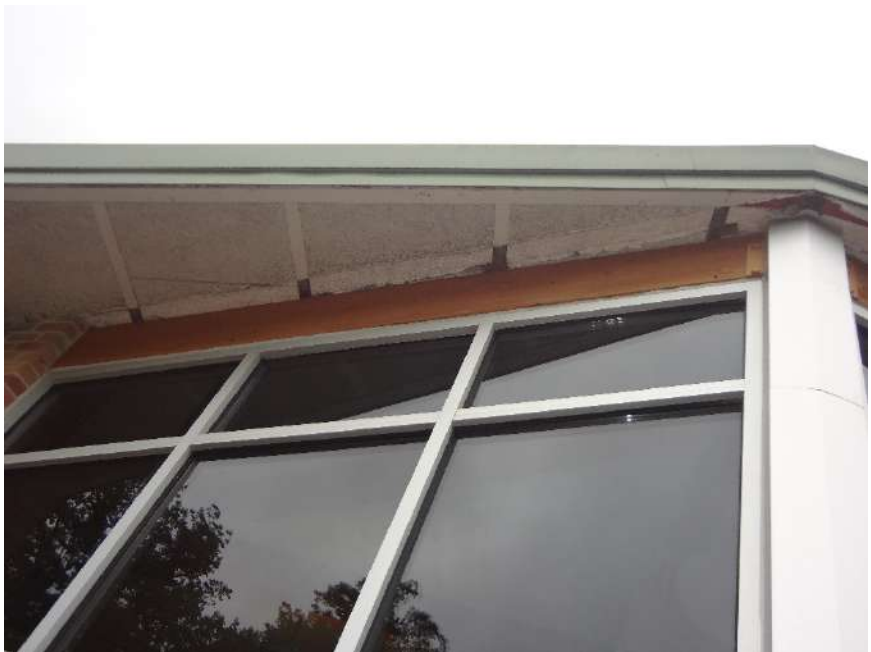
33. MISSING TRIM AT TECTUM SOFFIT EXPOSING STRUCTURE TO CORROSION + INFILTRATION - REPLACE METAL SOFFIT TRIM AND ENSURE OPENING IS WEATHER TIGHT
