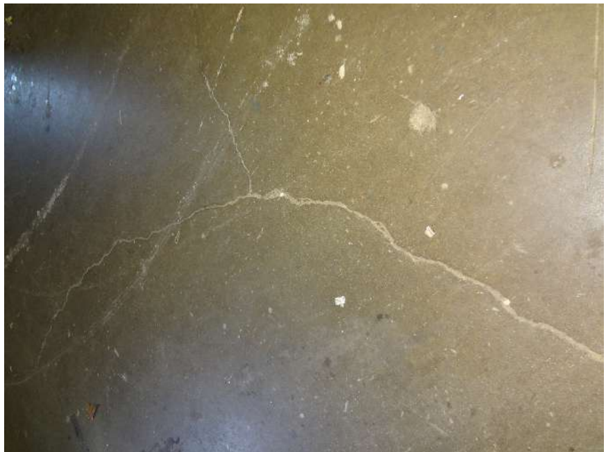
27. CRACKING IN CONCRETE FLOOR THROUGHOUT STORAGE AREA - CRACKING IS INHERENT IN CONCRETE. MONITOR FOR MOVEMENT, FINISH IF DESIRED
