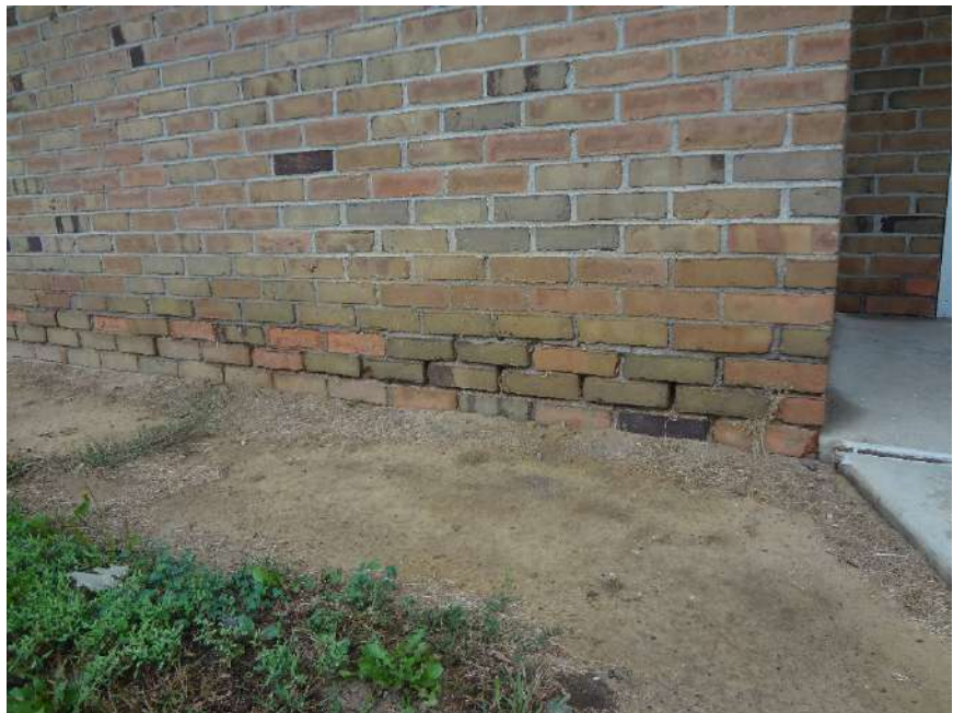
8. BROKEN + ERODED GROUT, 2'-0" ABOVE GRADE AND BELOW, TYPICAL - CLEAN & REPOINT MASONRY AS NEEDED FOR DAMAGED JOINTS. INSPECT ANNUALLY.
