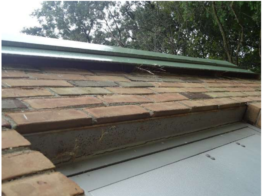
31. WIDE OPENING AT METAL ROOF FLASHING ALLOWING WEATHER INFILTRATION + NESTING - CLEAN DEBRIS FROM OPENING AND INFILL FLASHING TO CLOSE AREA OF INFILTRATION
