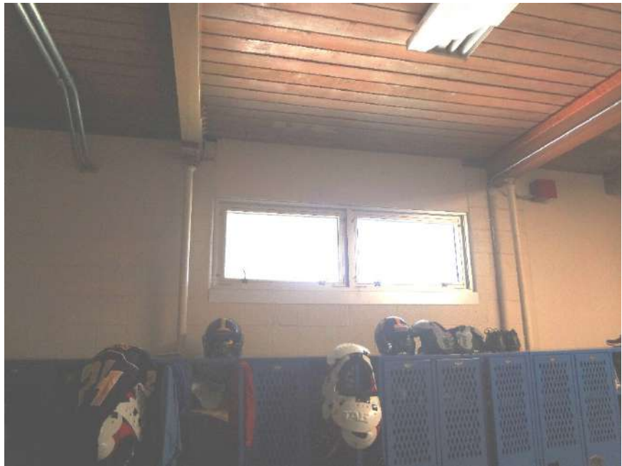
22. TWO RETROFIT STEEL JACKPOSTS AT LAMINATED WOOD BEAMS - CONSULT STRUCTURAL ENGINEER. TO BE REPAIRED/REPLACED DURING 2019 REMODEL
