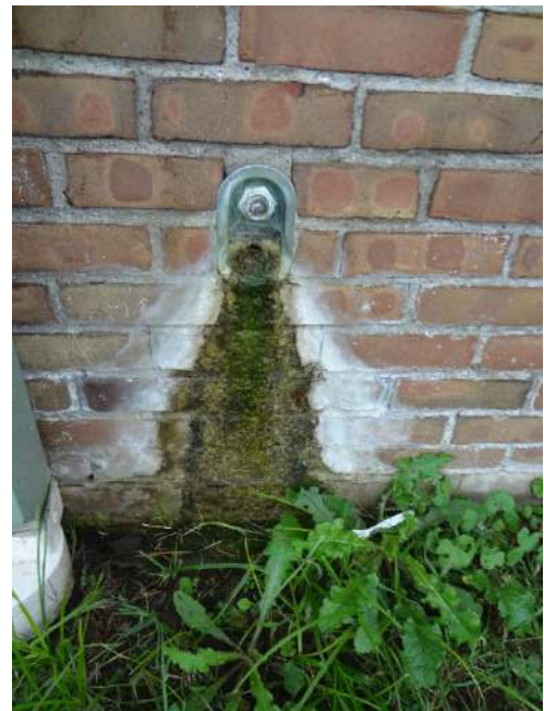
12. ORGANIC GROWTH + STAINING BELOW BROKEN WATER BIB - CLEAN ORGANIC MATTER FROM BRICK, INSPECT WATER BIB AND REPAIR AS REQUIRED
