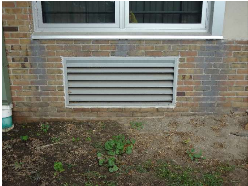
7. ALUMINUM STAINS ON BRICK, TYPICAL AT ALL WINDOWS THROUGHOUT FACILITY - CLEAN AND SEAL MASONRY AS NEEDED IN ALL SIMILAR LOCATIONS.
