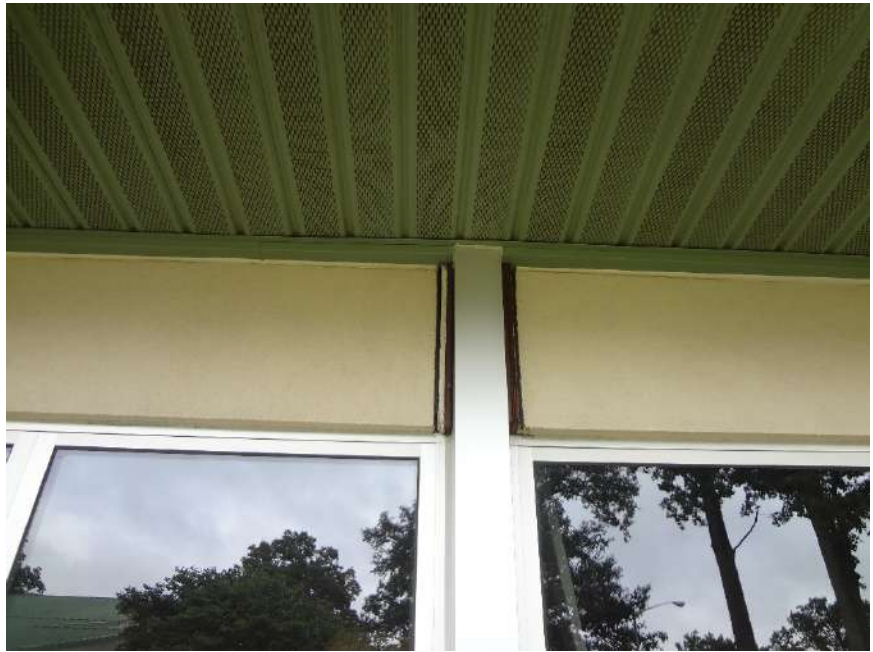
9. PLYWOOD + GYPSUM BOARD EXPOSED TO EXTERIOR ELEMENTS - CUT-BACK PLYWOOD AND GYPSUM, INFILL OPENING FOR WEATHER TIGHTNESS
