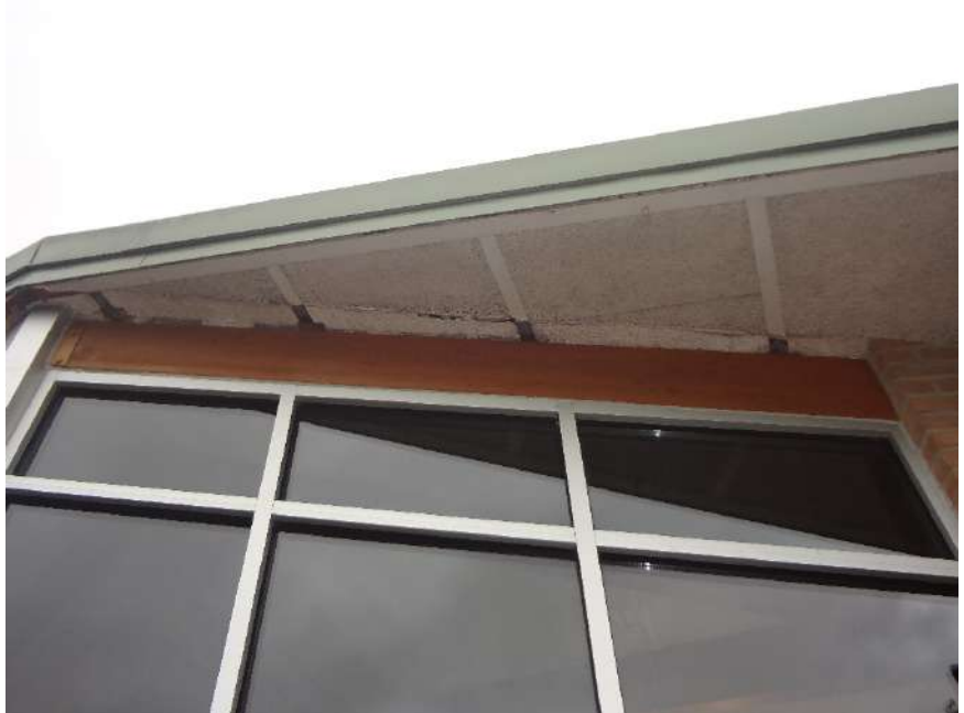
32. MISSING TRIM AT EAVE SOFFIT EXPOSING STRUCTURE TO CORROSION + INFILTRATION - REPLACE METAL SOFFIT TRIM AND ENSURE OPENING IS WEATHER TIGHT
