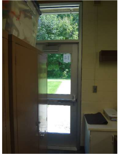
39. MISSING BACKER ROD + SEALANT AROUND ENTIRE DOOR FRAME - INSTALL BACKER ROD AND CAULK AROUND FRAME, INSPECT WEATHERSTRIPPING
