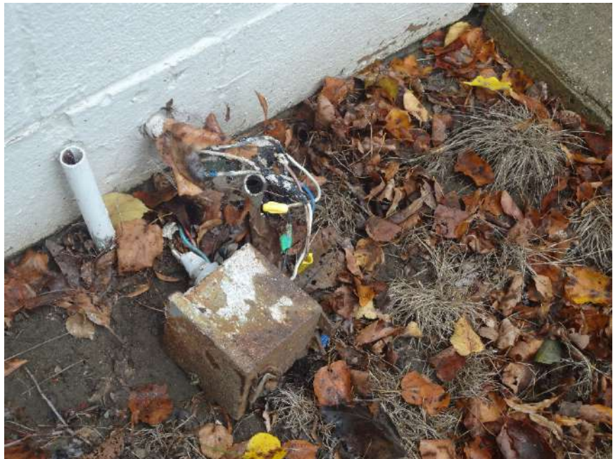
11. BROKEN CONDUIT + EXPOSED WIRING OF ABANDONED JUNCTION BOX - DISCONNECT JUNCTION BOX AND CAP ELECTRICAL AS REQUIRED
