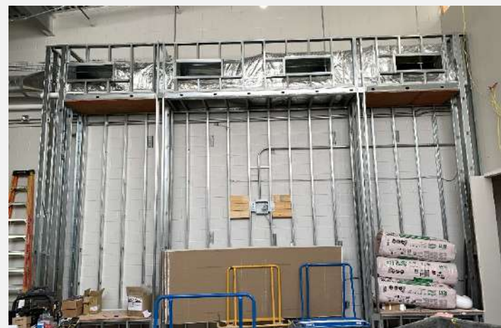
Phase 2 Addition: Main Lobby
