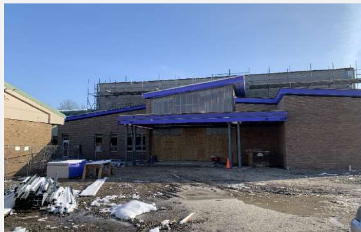
Phase 2 Addition: Multi-Purpose Gym Entry
