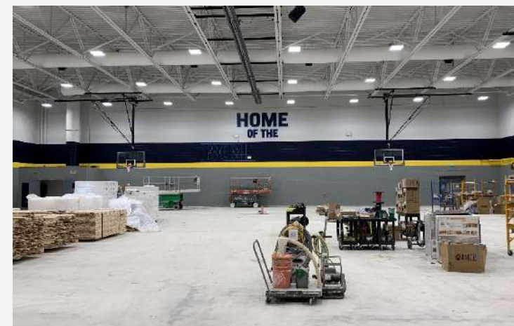
Phase 2 Addition: Multi-Purpose Gym
