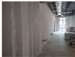
Above: Room 220 Mudding and Taping
