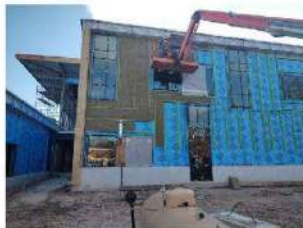
Above: Installing insulation on North side.
