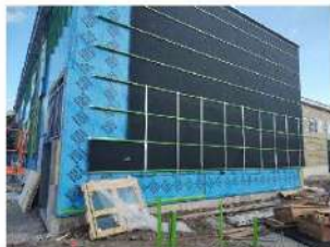
Above: Installed reinforced black insulation on Northwest corner wall.
