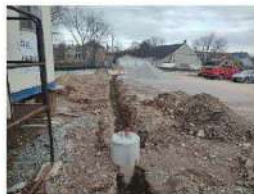
Above: Trenching for electrical conduit for Light Poles.
