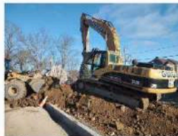
Above: Excavating bioretention area.
