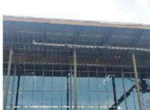
Above: Work on framing exterior soffit detail on the east side of the building.
