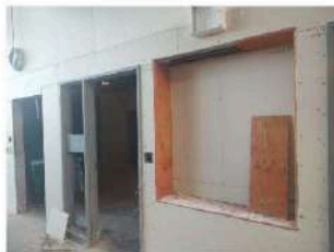
Above: Framing in display case in the main entrance Foyer.
