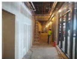
Above: Taping in corridor C102.
