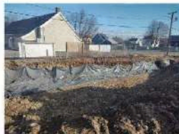
Above: Lining placement for retention area.
