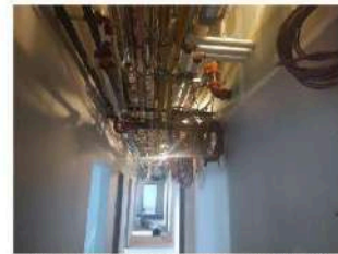
Above: Continuing to hang data lines in corridor C102 and run inter duct.
