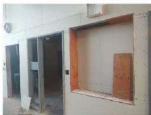
Above: Framing in display case in the main entrance Foyer.
