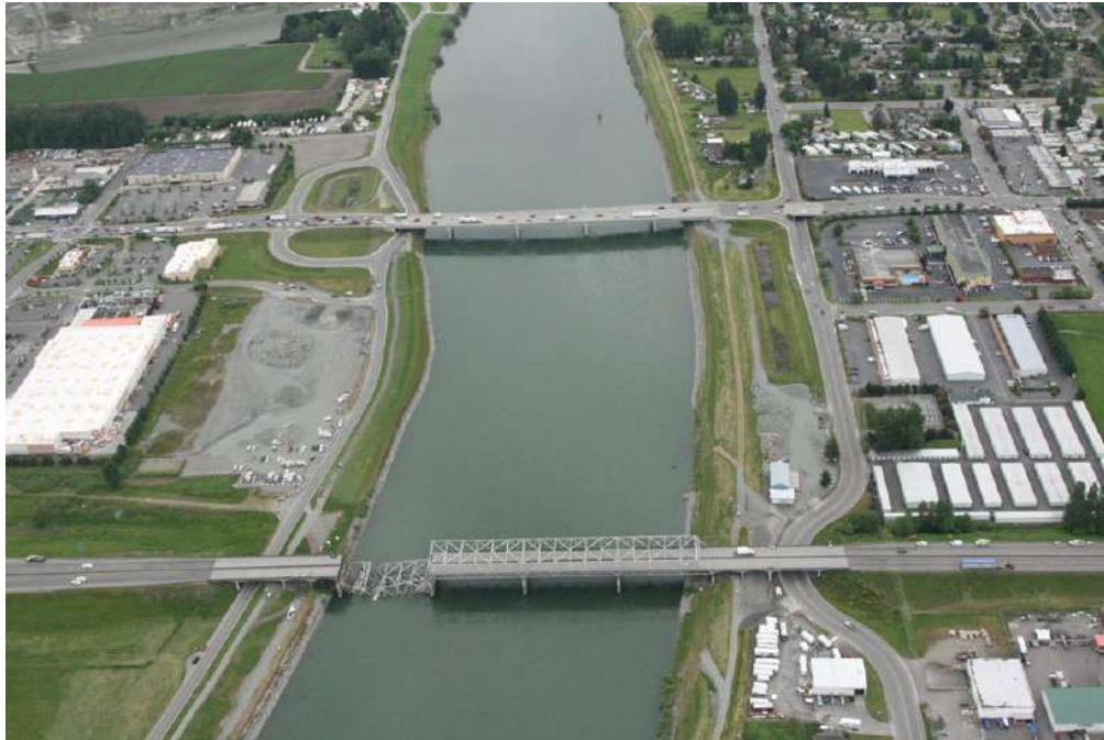
Figure 3-9 Extended View of Skagit County Bridge Collapse
