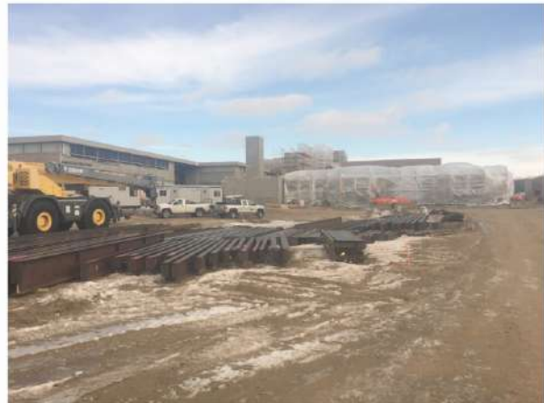
Structural Steel Delivered and Staged – West View of New South Classrooms
