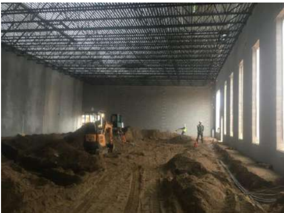
New Weight Room Roofed In and Underground Electrical Being Installed
