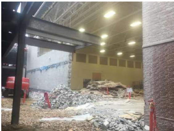
Existing Competition Gym Exterior Wall Demolition
