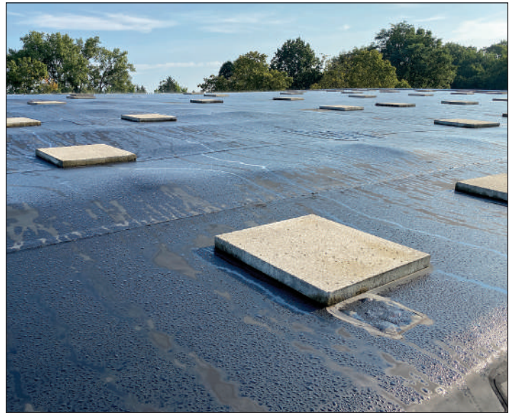
Delaminated Areas of Gym Roof
