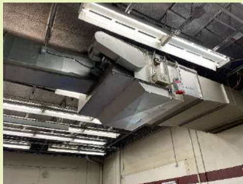
Goffstown High School T8 Lighting
