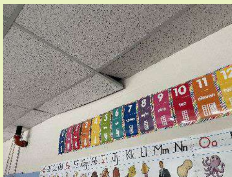
Maple Avenue Elementary Ceiling Tiles with Large Gap
