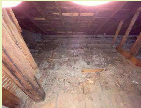
SAU Office Attic Insulation
