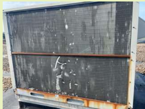
Mountain View Middle School Roof Top Unit in Poor Condition
