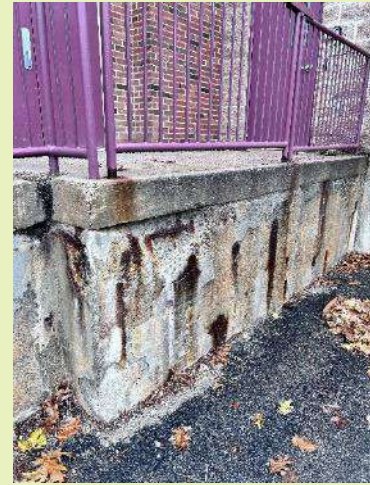
Goffstown High School Loading dock area concrete in need of repairs
