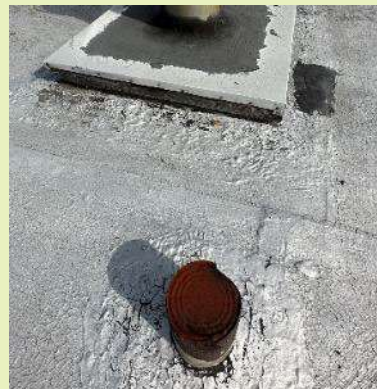
Bartlett Elementary School Upper Roof
