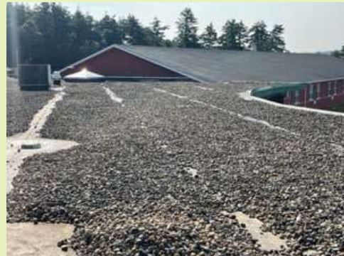
Mountain View Middle School Roof Section
