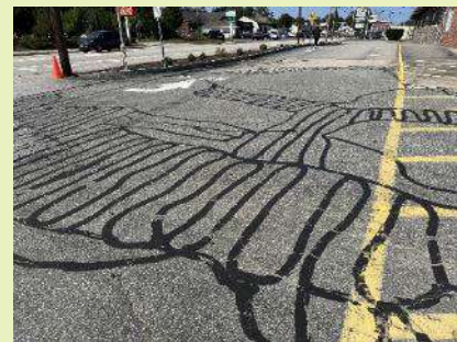
Bartlett Elementary School Parking Lot
