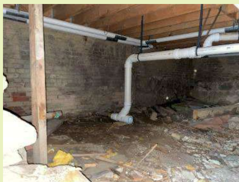
SAU Office Basement Conditions
