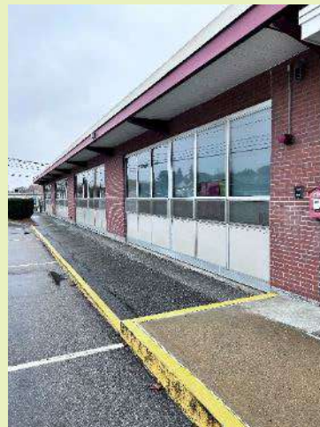
Bartlett Elementary Front Windows
