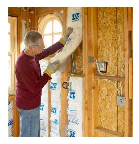
Next, the builders fill the empty spaces inside the walls and under the roof. This helps keep the house warm in winter and cool in summer.
