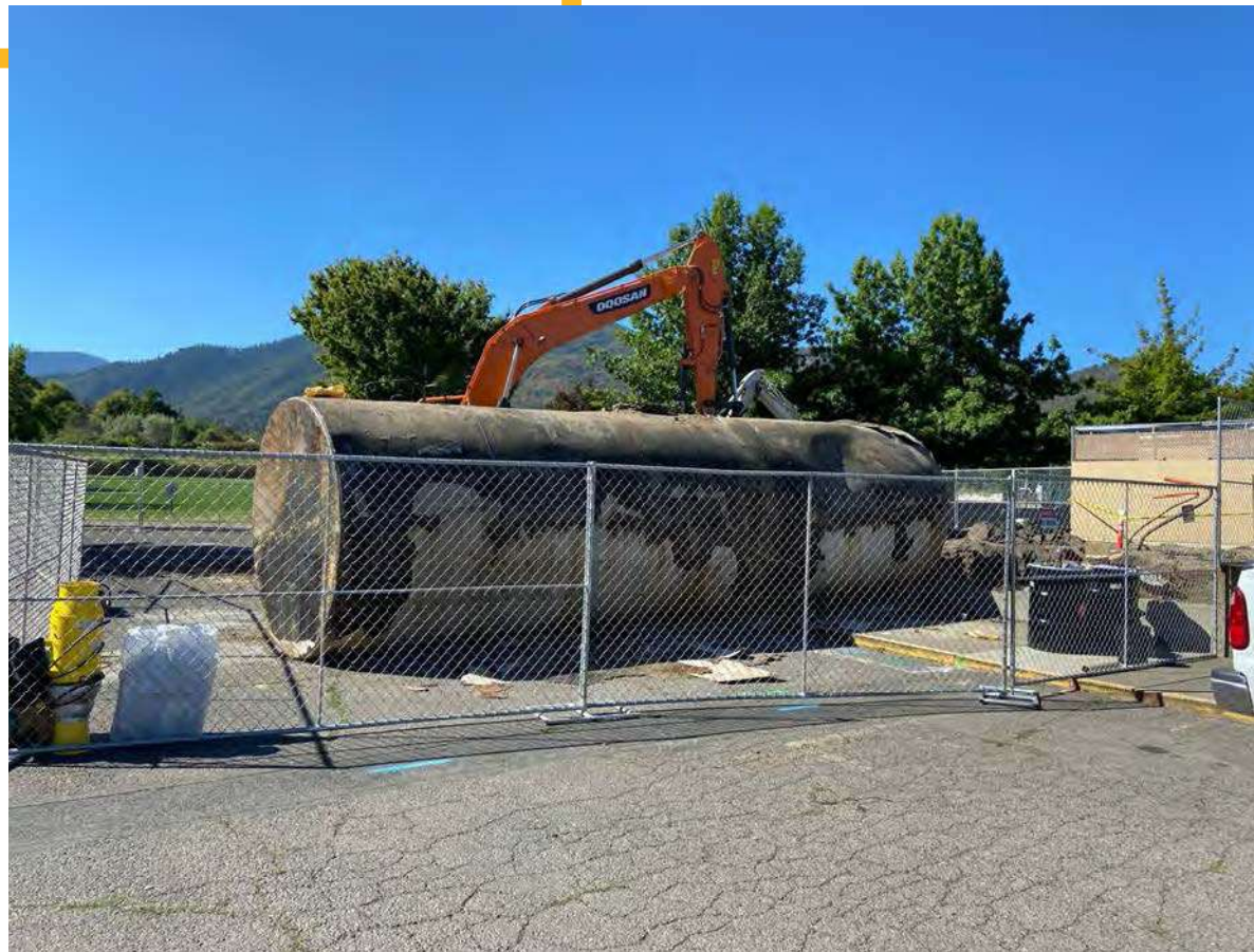
Diesel Tank Removal
