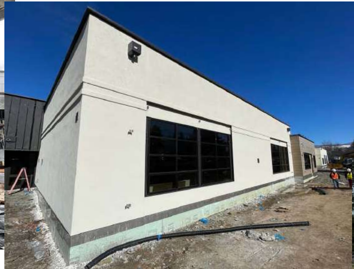
EXTERIOR CEMBRIT CLADDING AND NEW STUCCO ON THE SOUTH SIDE OF THE BUILDING
