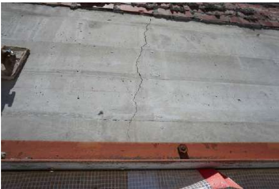
Figure 13: Fracture in concrete beam between ledger anchors
