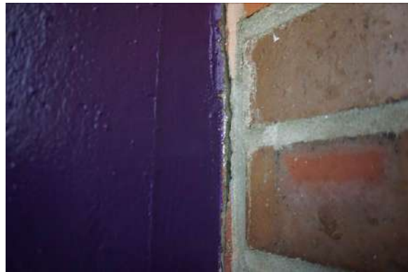
Figure 2: Separation in mortar joint at north concrete column/masonry wall interface
