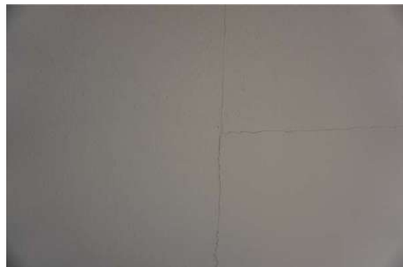
Figure 10: Separations in gypsum board ceiling finish at east end of south hallway
