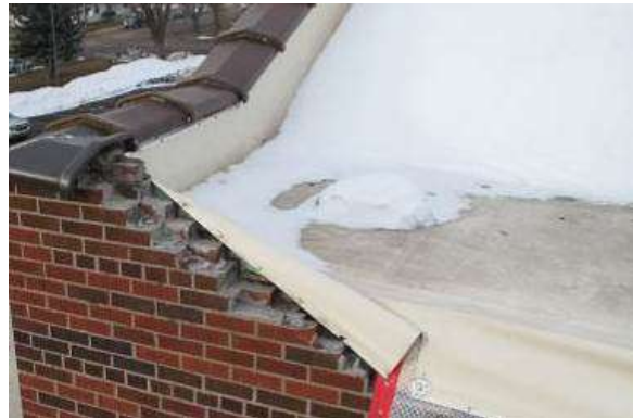
Figure 16: Tears in thermoplastic membrane at holes along south edge of membrane
