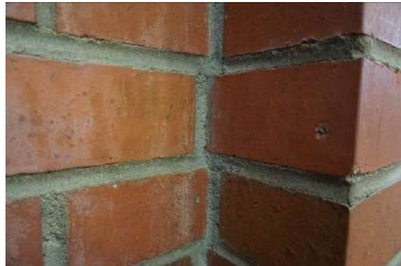
Figure 8: Condition of brick masonry column/adjacent wall interface opposite side of column shown in Figure 7
