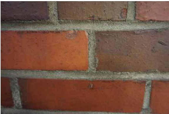
Figure 1: Isolated linear fracture in field of east masonry wall
