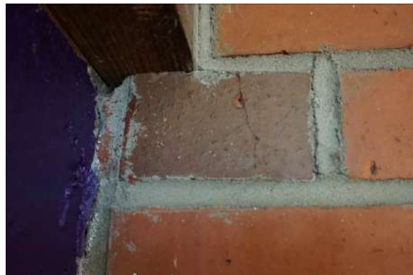
Figure 4: Isolated fracture in masonry brick adjacent to north concrete column
