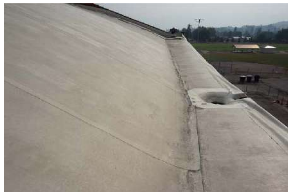
Figure 14: View of thermoplastic membrane at location of missing/collapsed parapet
