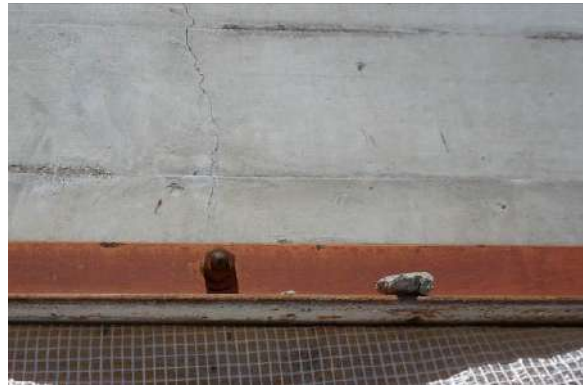
Figure 12: Vertical, discontinuous fracture in concrete beam coincident with ledger anchor
