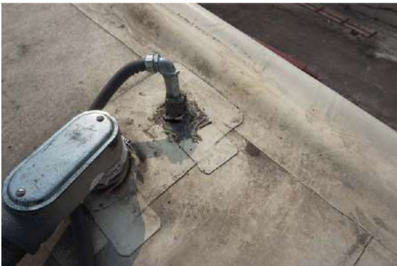
Figure 15: Condition of thermoplastic membrane at pipe penetration at roof edge shown in Figure 14
