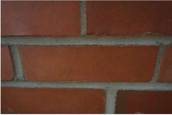
Figure 5: Discontinuous/isolated separation in horizontal mortar joint below east window in north masonry walls
