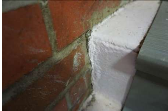
Figure 6: Discontinuous separation at interface of concrete stair/masonry wall at southeast corner of gymnasium
