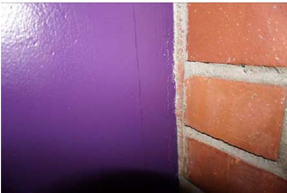
Figure 3: No separation in mortar joint directly below separation shown in Figure 2
