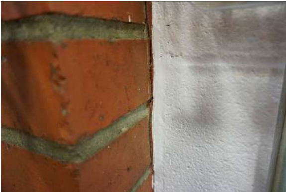
Figure 7: Separation at interface of brick masonry column/CMU wall
