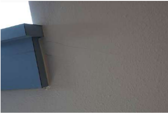
Figure 11: Isolated diagonal fracture in wall finishes at bottom right-hand corner of south-facing music room window
