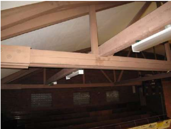
Figure 19: Checking in bottom chord of fourth truss from east wall
