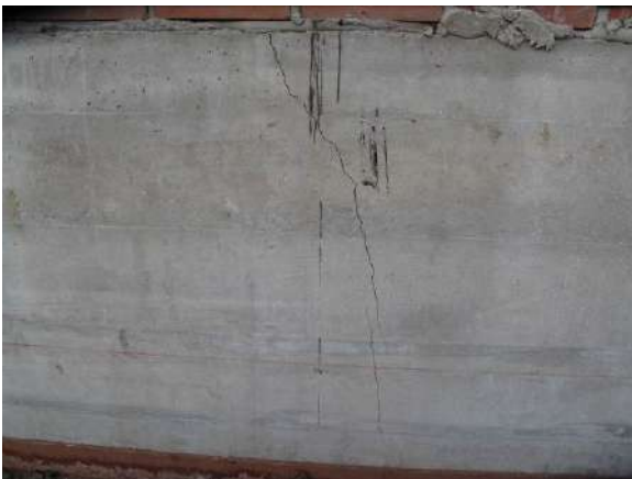
Figure 9: View of fracture in exposed beam near east end of south gymnasium wall
