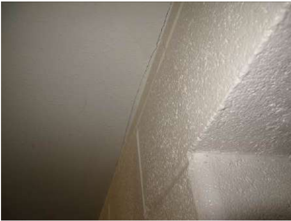
Figure 13: Fracture in ceiling finishes adjacent to showers of northwest locker room
