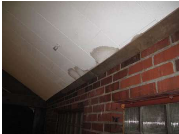
Figure 20: Moisture-stained ceiling tiles along south gymnasium wall
