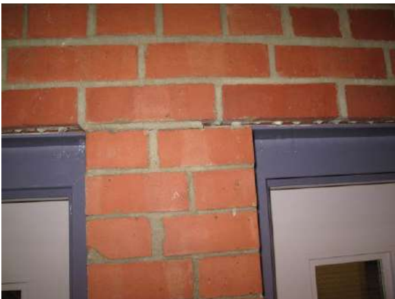
Figure 15: Separations at lintel/masonry interface of south doorways, west gymnasium wall
