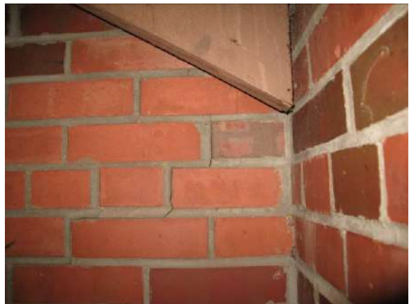
Figure 16: Stair-step mortar joint separations at east wall, southeast corner of gymnasium
