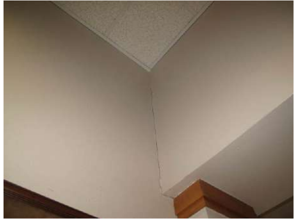
Figure 12: Wall-to-wall separation at west library wall
