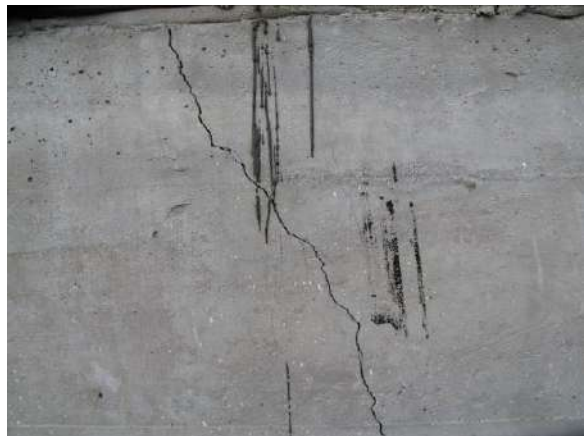
Figure 10: Closer view of top portion of fracture shown in Figure 9
