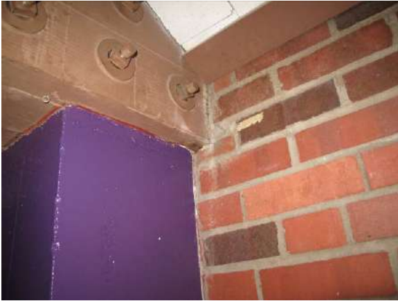
Figure 17: Unpainted wood at south end of truss bottom chord, first truss from east gymnasium wall
