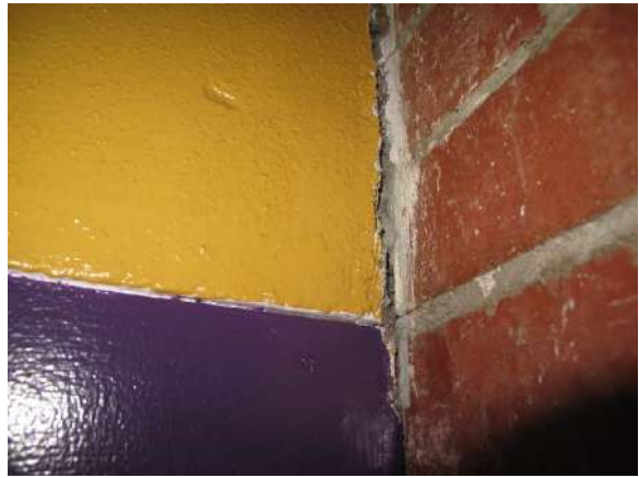
Figure 14: Separation at concrete column/masonry wall interface, southwest corner of gymnasium
