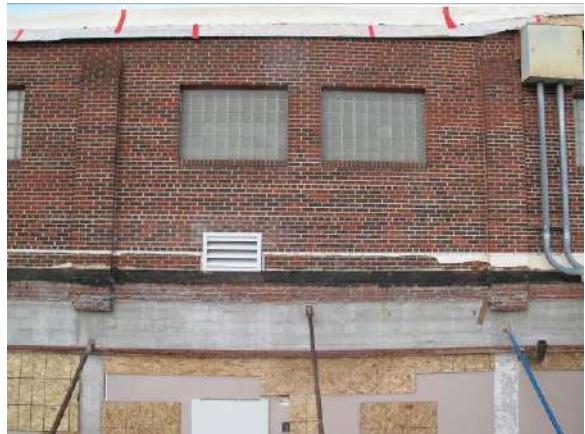
Figure 8: Exposed concrete columns and beam near southeast corner of gymnasium
