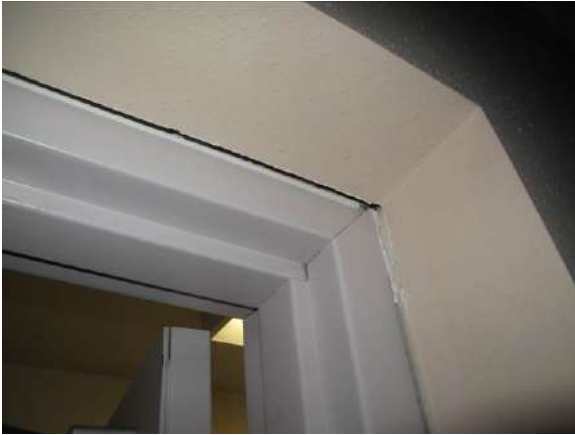
Figure 11: Separation at door frame/wall interface at doorway to southeast classroom
