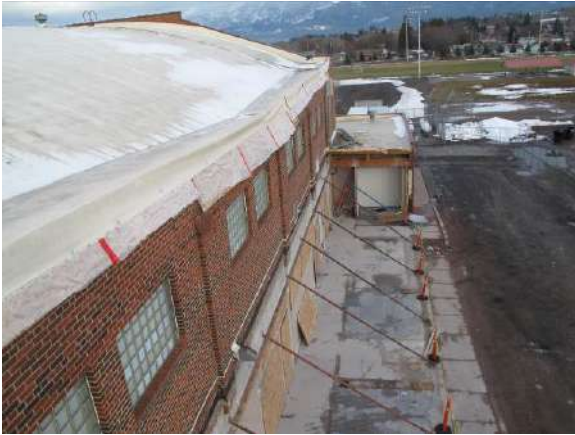
Figure 5: Missing portion of structure at south side of gymnasium
