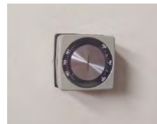
Typical Pneumatic Thermostat
