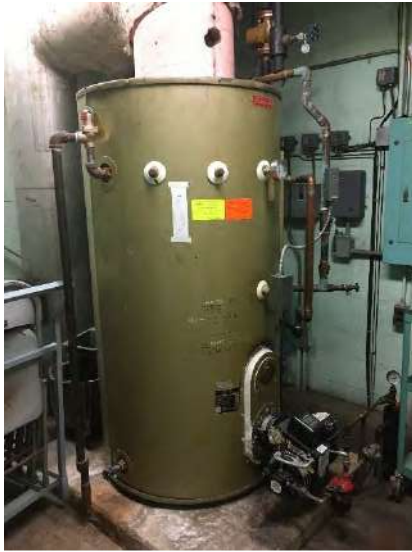
Oil fired water heater
