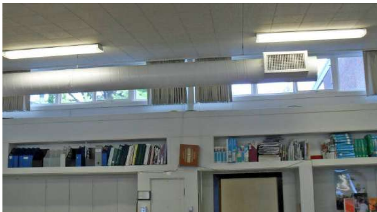
Typical Classroom Clerestory Windows blocked by ductwork
