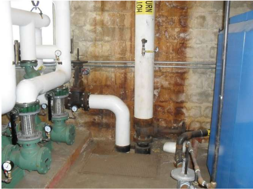
Figure 3 - HWS&R mains exiting the boiler room feeding Coffin
