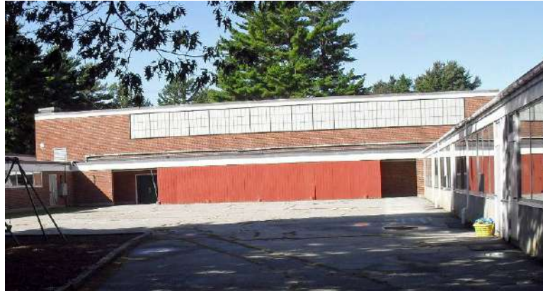
Exterior of Gym (Note infill storage with plywood siding)
