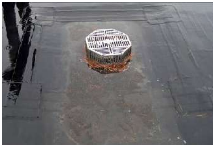
Typical roof drains set in sumps
