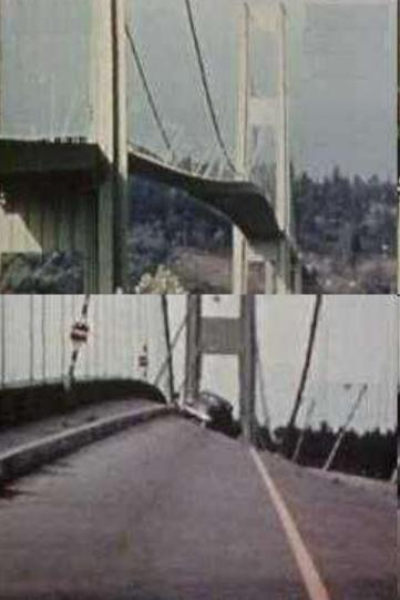
This photograph shows the twisting motion of the centre span just before the structure failed..
