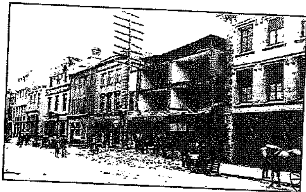
Figure 2. Earthquake damage to building on the south side of Broad Street, Charleston.
