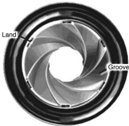
Figure 2.2.1 View of right hand twist rifling, showing lands and grooves.
