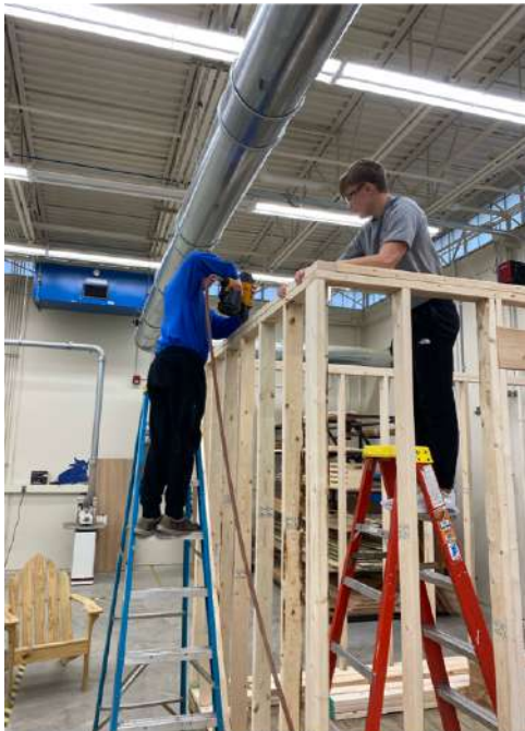
Malachi Peckham & Treyce Rollene putting on the top plate.
