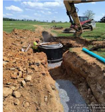
4" Force Main Manhole Installation
