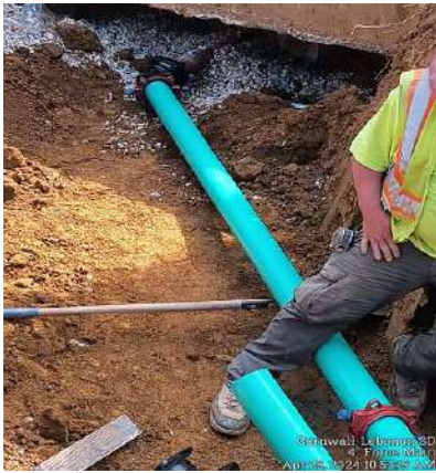
4" Force Main Connection To Pump Station
