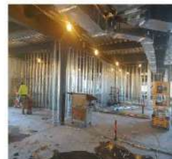
Above: Framing interior walls
