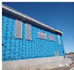
Above: Installed temporary window coverings to window openings until glass is delivered
