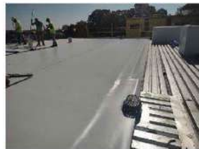
Above: Single Ply roofing on Pre-K, Gray
