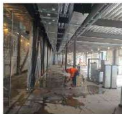
Above: Laying out rooms and installing wall track (mounting system)
