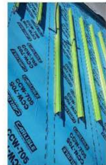
Above: Installing air and vapor barrier to Pre-K exterior walls
