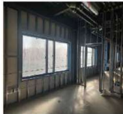
Above: The building is closed up for temporary heating
