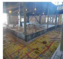
Above: Forming up transition between Pre-K and the Main Bldg.
