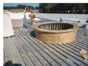
Above: Framing for skylight
