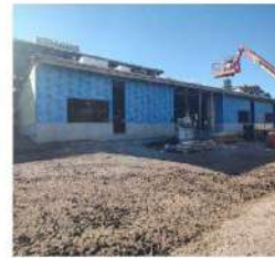
Above: Installing air and vapor barrier to Pre-K exterior walls
