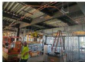
Above: Ductwork installation Level 2
