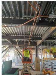
Above: Installing condensate lines
