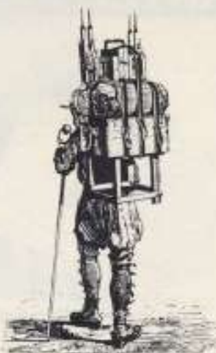
A Portable Darkroom of the 1860s. The darkroom of this period had to be set up close to the camera so the plate could be coated, loaded into the camera, and returned to the darkroom for development after the exposure and before the emulsion dried.
