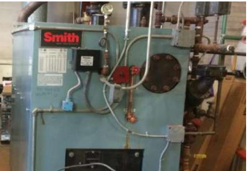
Ashaway School gas fired boiler system has reached its life expectancy and needs replacement.
