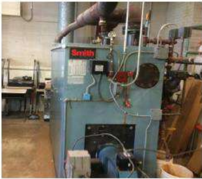
Ashaway heating steam gas fired boiler plant has reached its life expectancy and needs to be replaced
