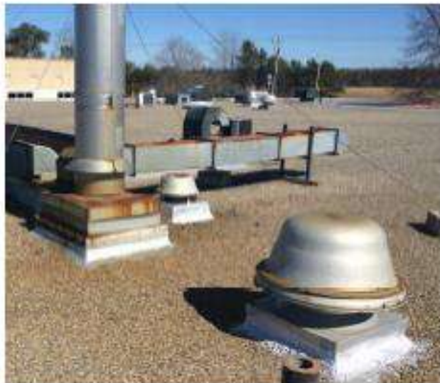
CHARIHotech Built-Up Roof System is past its life expectancy and needs to be replaced.
