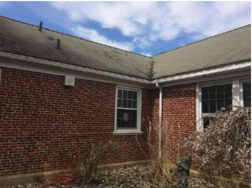
Replace asphalt shingle roof at Richmond Elementary School
