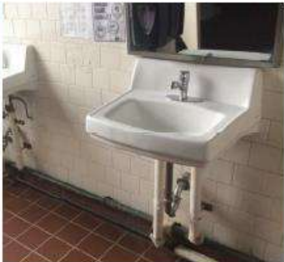
Richmond original plumbing fixtures should be replaced with ADA compliant fixtures and upgraded finishes.
