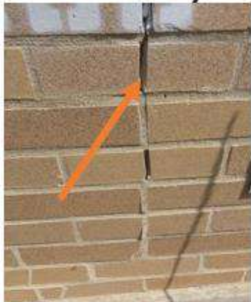
Charlestown brick and mortar cracking/missing at several locations. Brick should be repointed.
