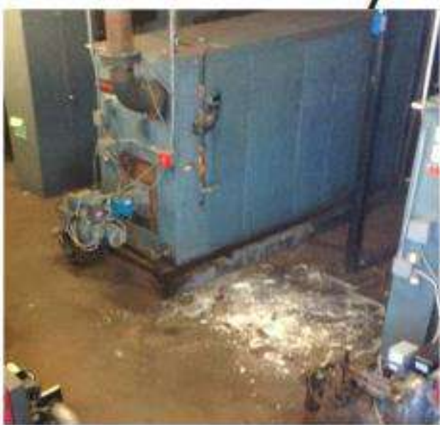
Charliho High School Heating hot water oil fired boiler reached life expectancy and is need of replacement.
