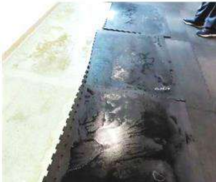
Chariho Middle School has signs of water ingress at several locations throughout the building. Exploratory analysis/repair is needed.
