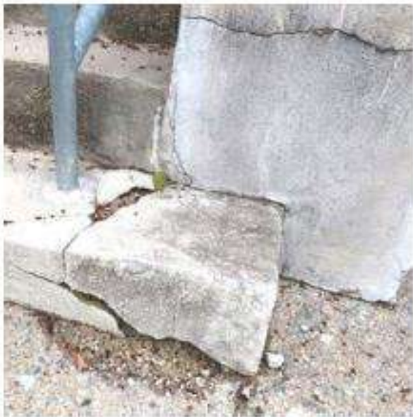
Hope Valley concrete stairs are deteriorating and should be replaced.
