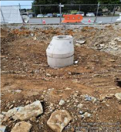
New Sewer Manhole on Building Pad
