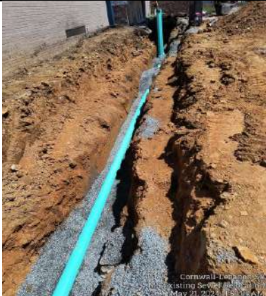
New Middle School Sewer Installation
