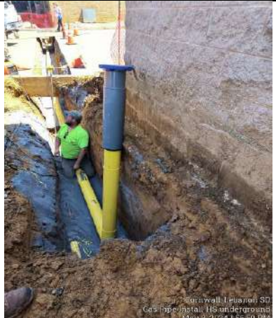
New Underground Gas Line Rear Of High School
