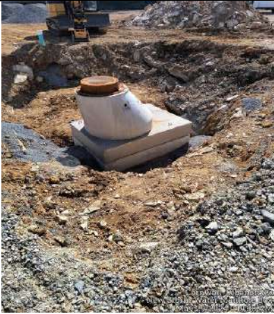
New Storm Water Manhole
