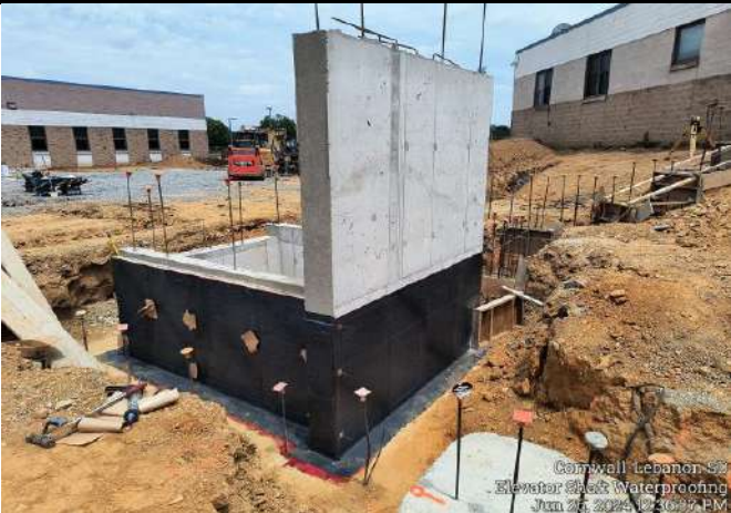
Elevator Shaft Wall and Pit with Waterproofing
