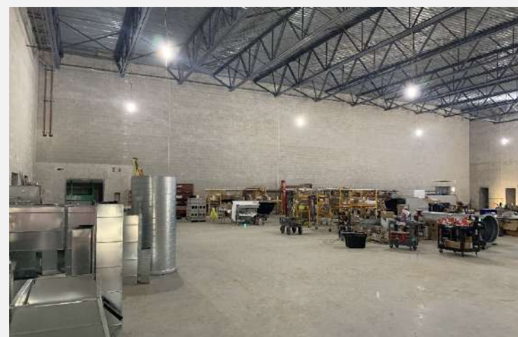
Phase 2 Addition: Multi-Purpose Gym
