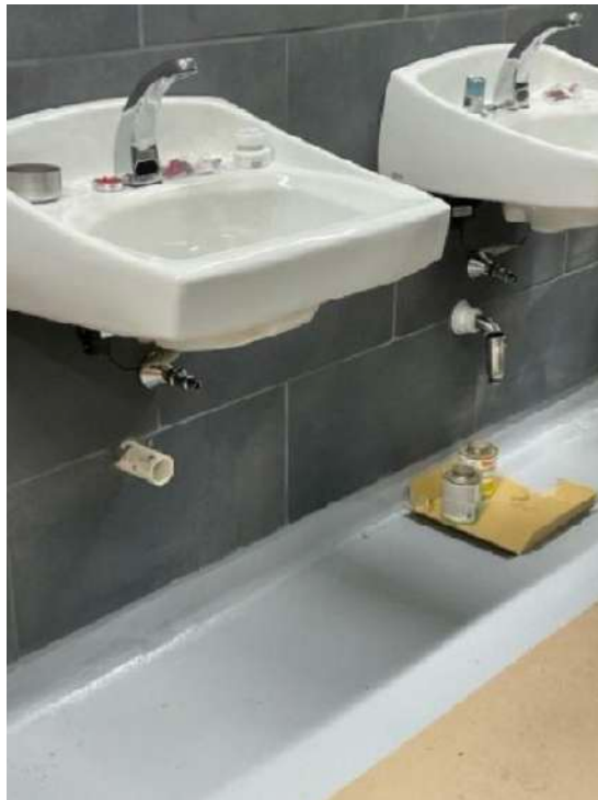
Installation of Sinks In Boys' Restroom
