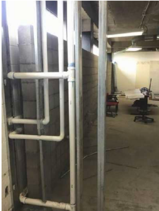
New Plumbing Installed
