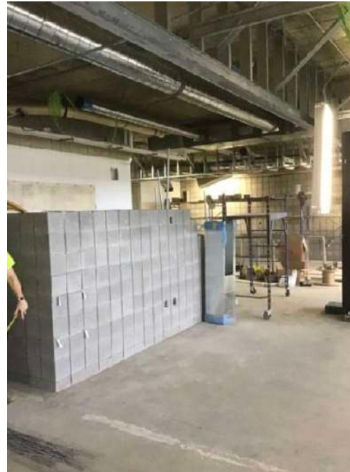
New CMU Block Wall
