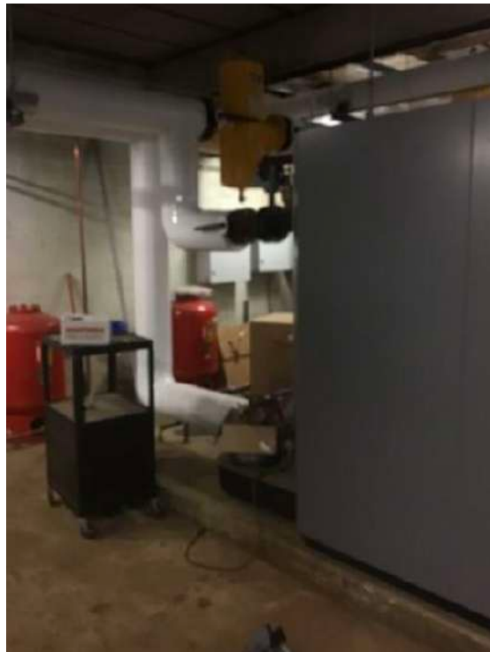
Insulation of Pipes in the Boiler Room
