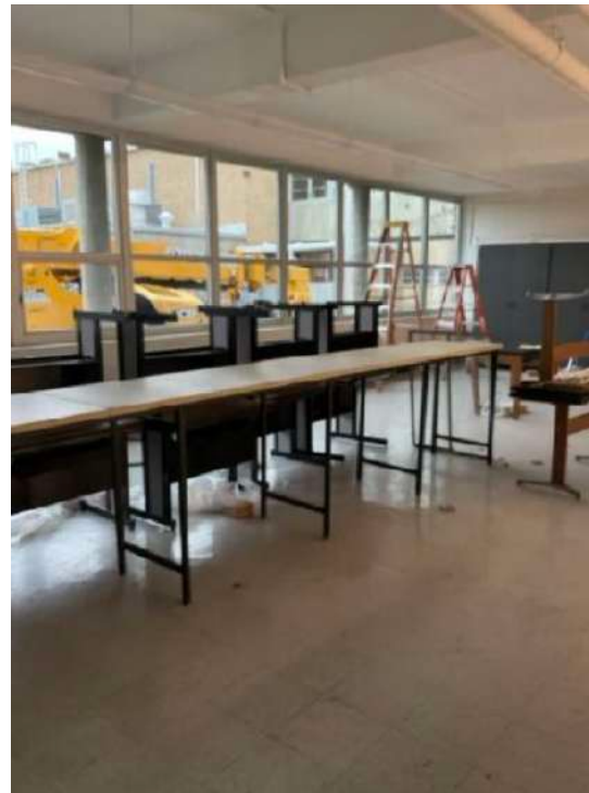
Installation of Classroom Windows
