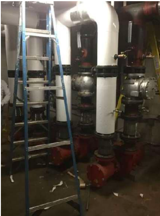
Insulation of Pipes in the Boiler Room
