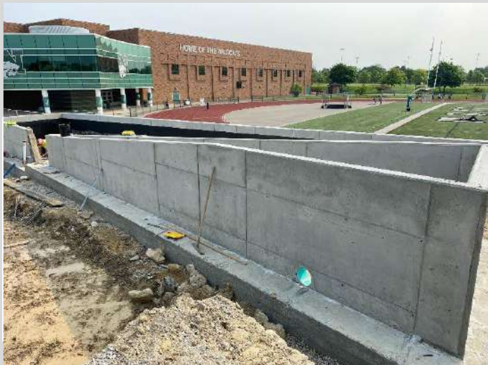
Ramp Foundation Walls
