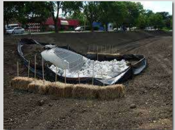
End Section Replacements
