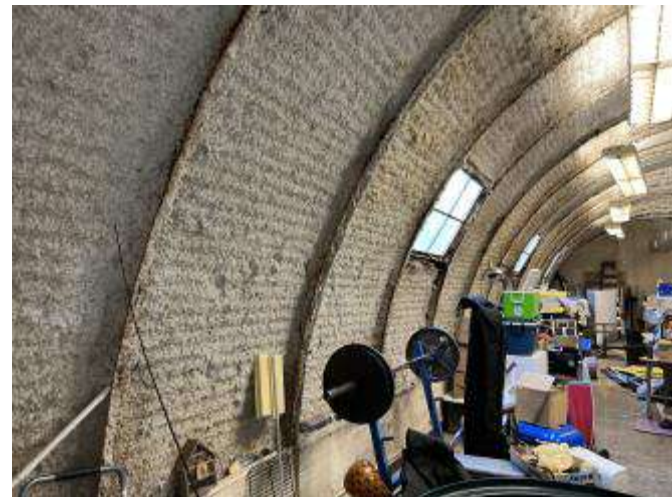
Photo 12: (HA-12) Quonset Hut Wall and Ceiling Insulation
