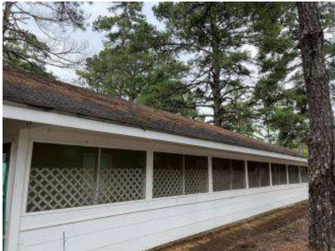
Photo 1: (HA-01) Main Building Roof Shingles with Felt
