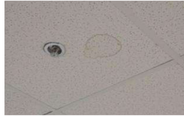
Existing water damaged ceiling tile
