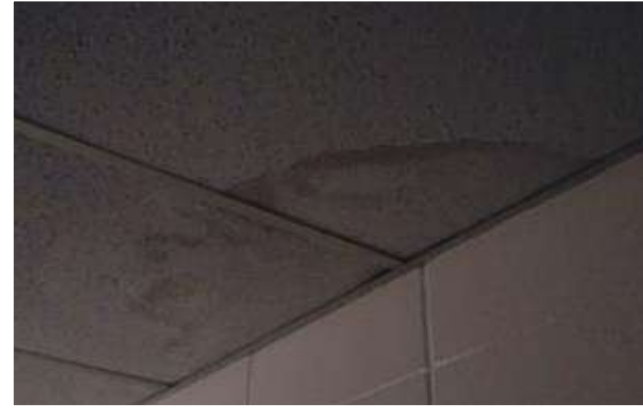
Existing water damaged ceiling tile
