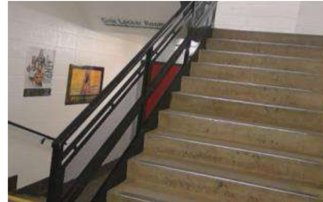
Existing non-compliant stair railings
