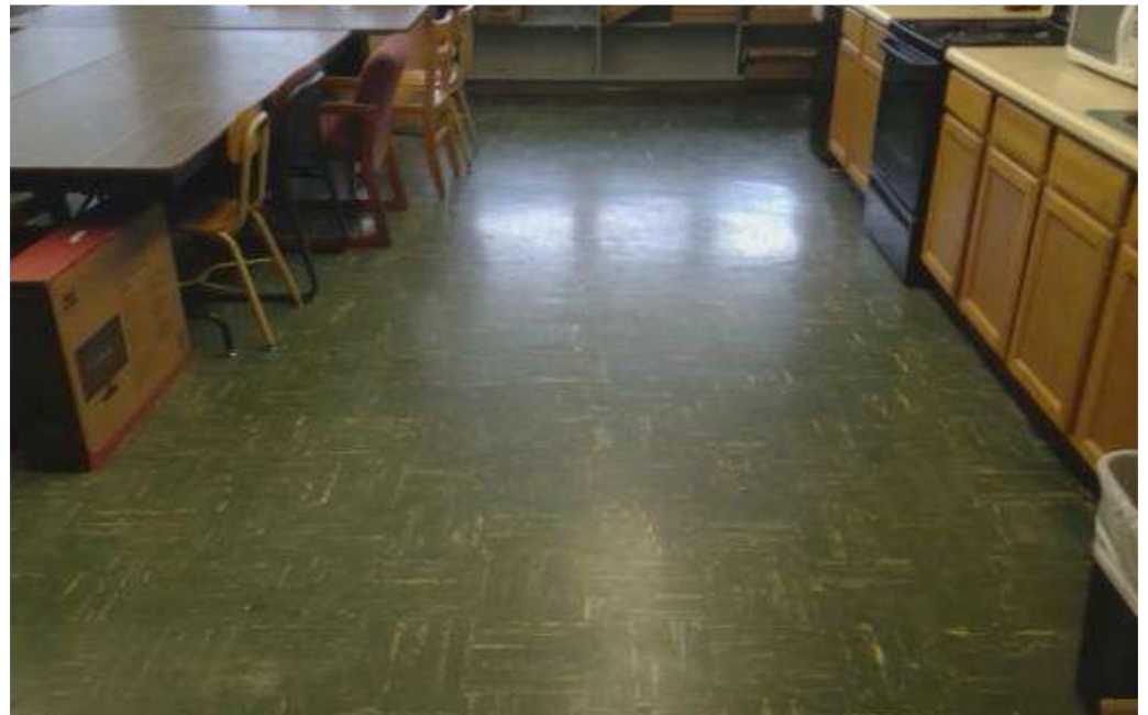
Existing asbestos containing floor tile
