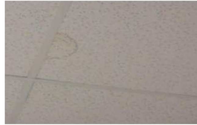
Existing water damaged ceiling tile
