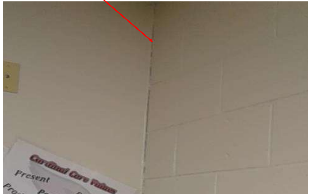
Existing masonry caulk joint
