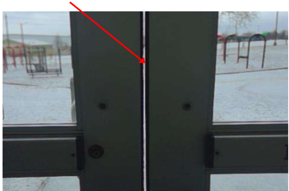
Existing air gap at exterior doors
