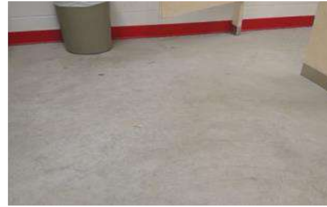
Existing sealed concrete floor
