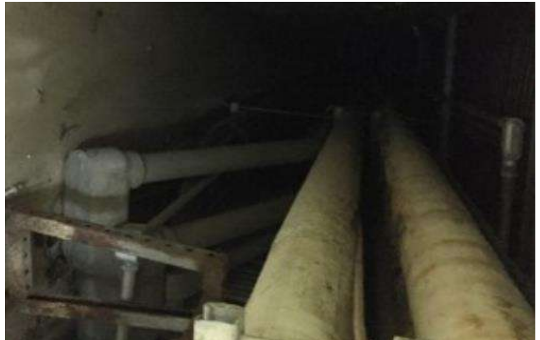
Existing asbestos insulation
