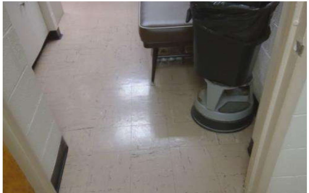
Existing asbestos containing floor tile
