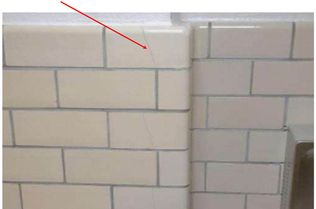
Existing crack in wainscoting
