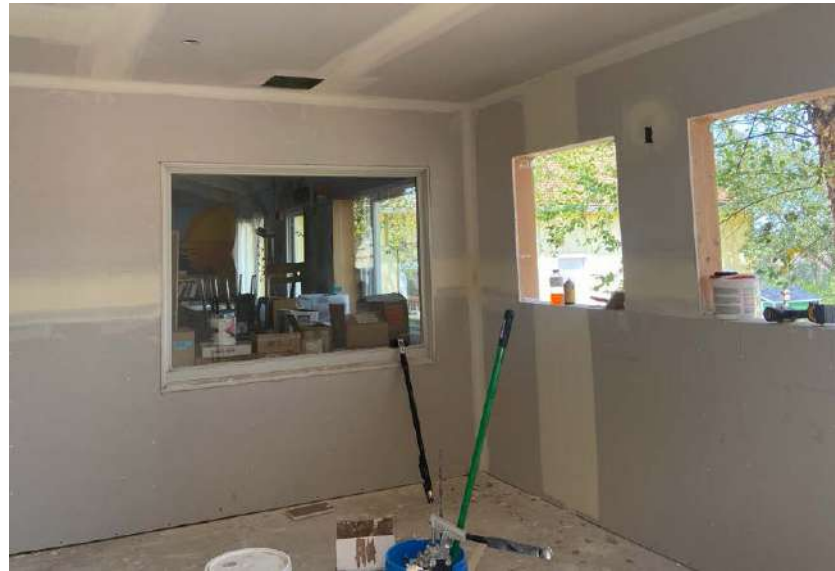
DRYWALL AT NEW HEALTH ROOM
