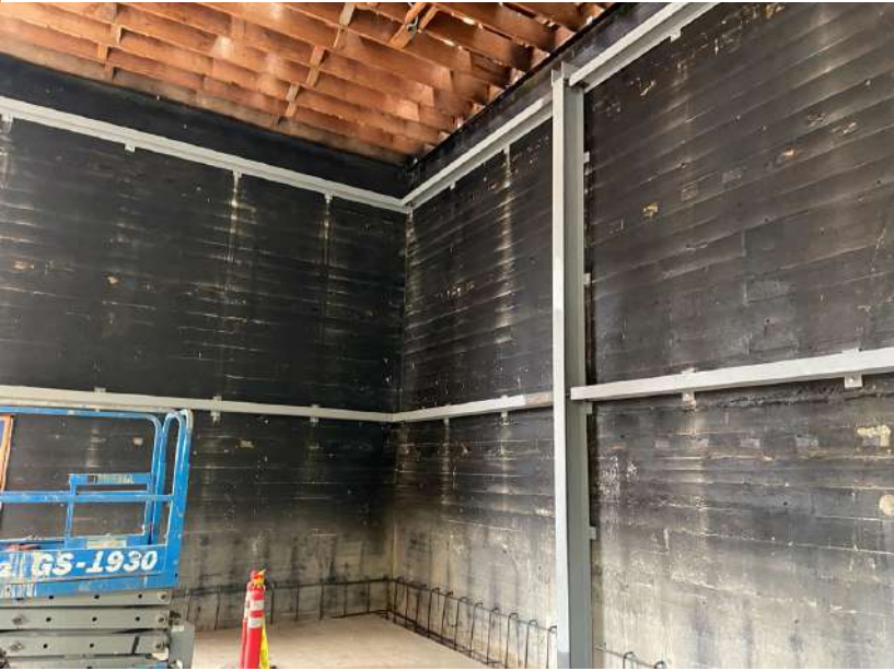
NEW STEEL STRONGBACKS IN CAFETERIA
