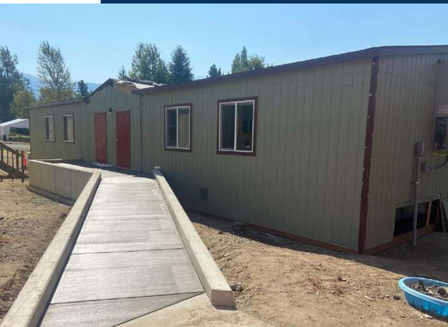
NEW MODULAR AND CONCRETE ACCESS RAMP
