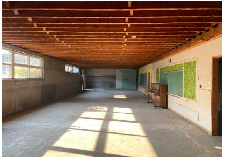
EXPOSED STRUCTURE IN BASEMENT
