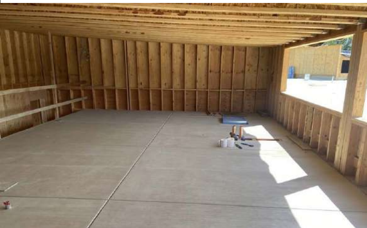
NEW MECHANICAL MEZZANINE
