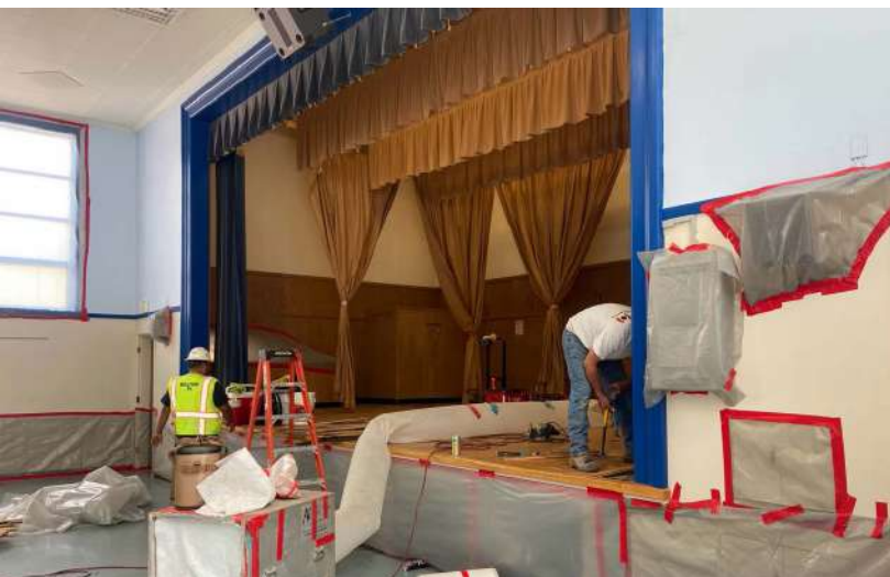
START OF ABATEMENT IN THE CAFETERIA
