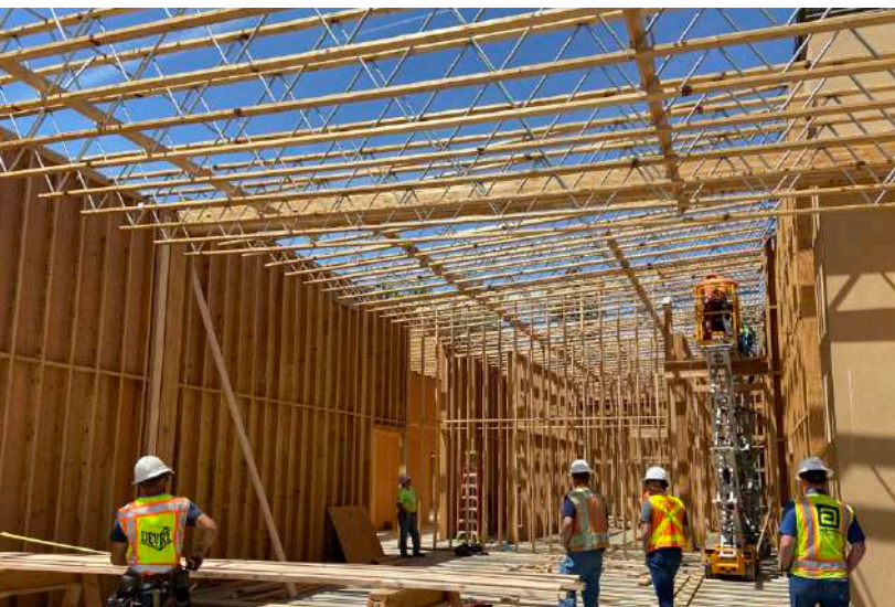
FRAMING AND STRUCTURAL STEEL AT THE NEW ADDITION
