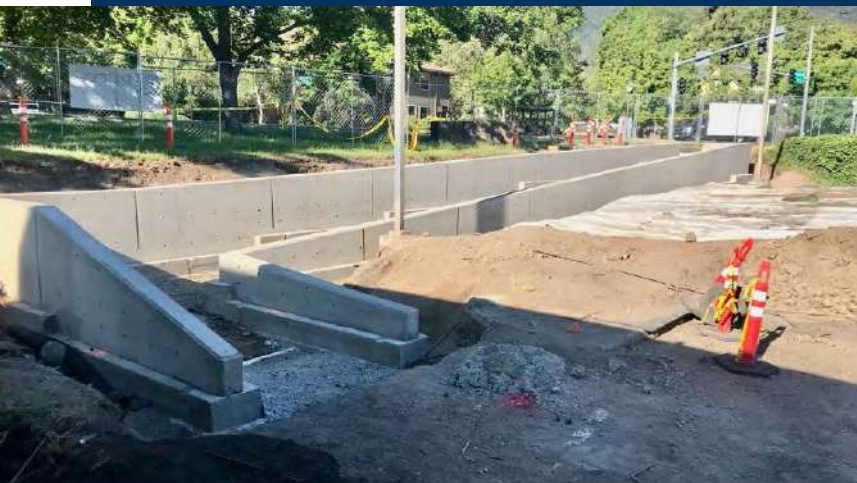
CONCRETE WALLS AND FOOTINGS AT SISKIYOU RAMP
