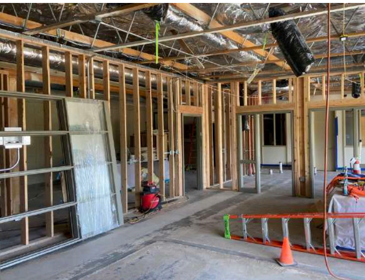
NEW FRAMING, ELECTRICAL ROUGH IN AND DOOR FRAMES IN THE ADMIN AREA
