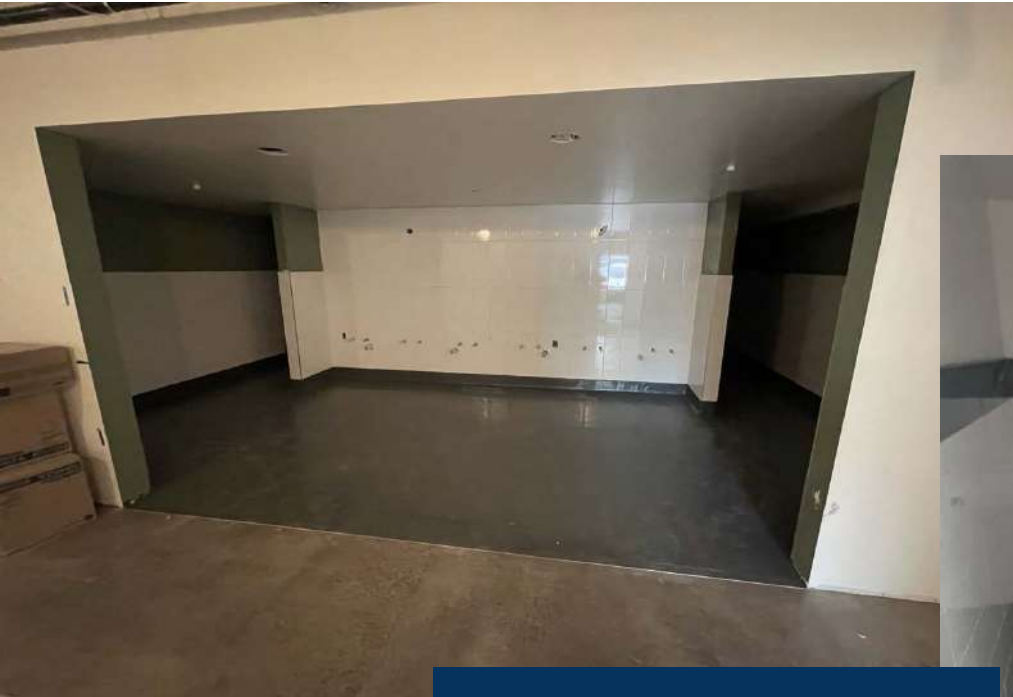
TRAILS: COMPLETED PAINT, TILE AND EPOXY FLOORING IN RESTROOMS
