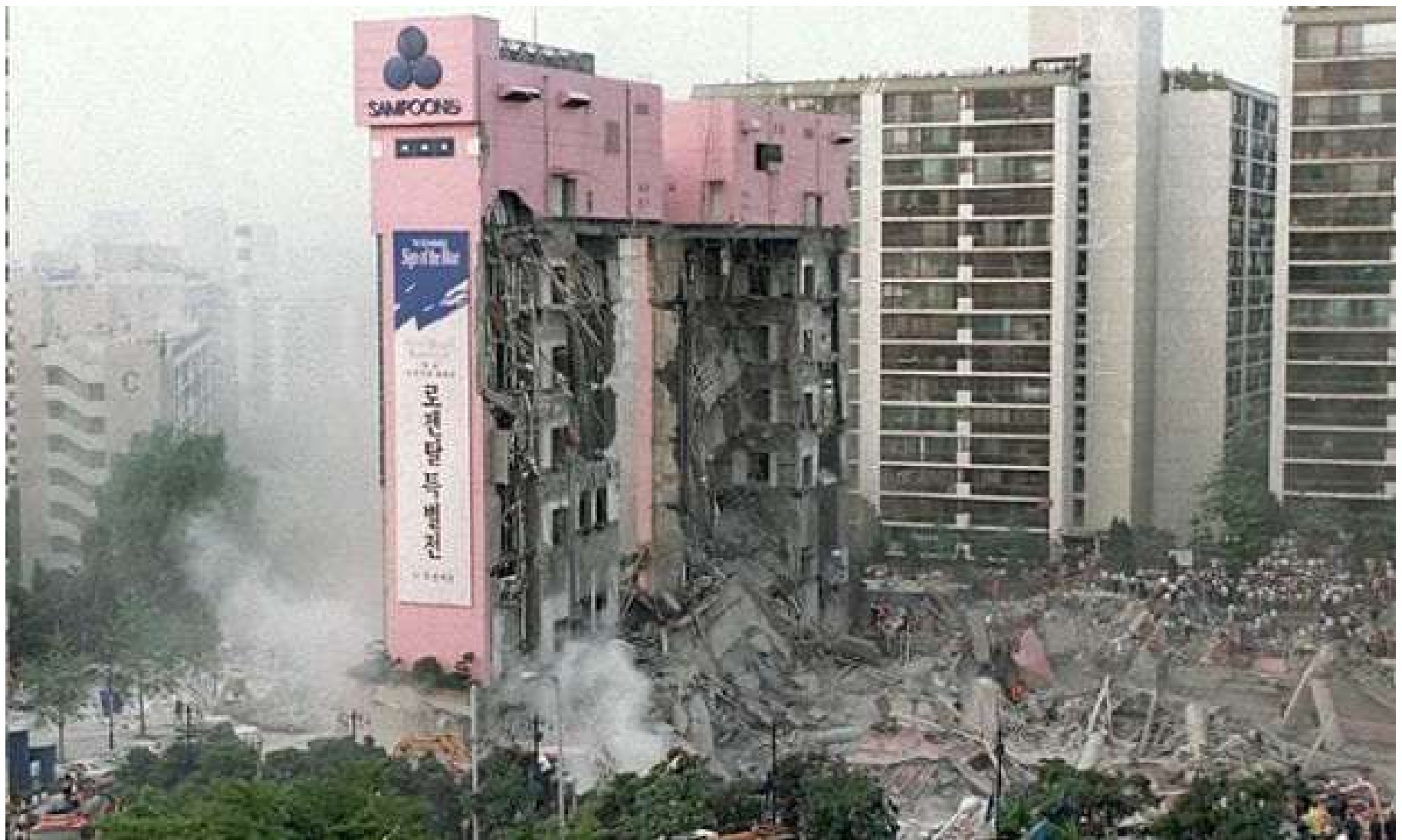
The remains of the Sampoong Department store on the 29 June 1995 just hours after it collapsed, when air conditioning units on the roof crashed through to the floor.
