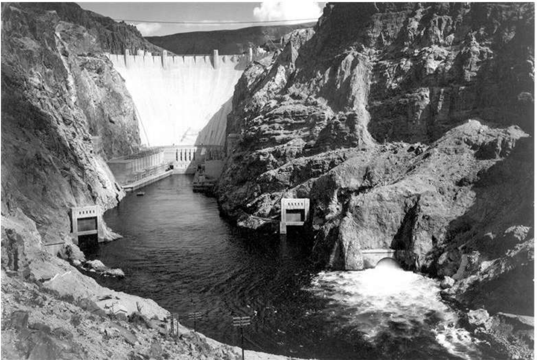
Hoover Dam, once known as Boulder Dam, is a concrete arch-gravity dam in the Black Canyon of the Colorado River, on the border between the U.S. states of Arizona and Nevada. When completed in 1936, it was both the world's largest hydroelectric power generating station and the world's largest concrete structure. It was surpassed in both these respects by the Grand Coulee Dam in 1945. It is currently the world's 38th-largest hydroelectric generating station. In this image: Hoover Dam by Ansel Adams (1942).
