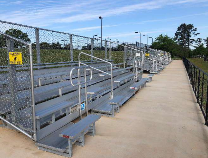
New concrete pad and bleachers at track.
