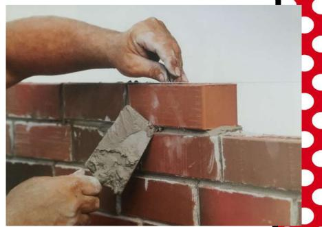
The bricklayer builds walls and houses using bricks. Bricks are made from clay--extremely fine, red soil that comes from the earth. A long time ago, people discovered that if you mixed clay with a little water, shaped it into a block, and then baked it in the hot sun, it would dry out and harden into a solid brick.
