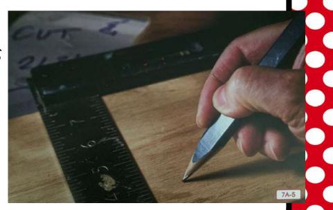
The carpenter makes a mark on the board with a pencil to show him where to cut. Carpenters have to be careful to get their measurements exactly right; otherwise, if they cut the wrong sized piece of wood, or cut it at the wrong angle, the piece will not fit together correctly and the house will not stand up properly up properly.
