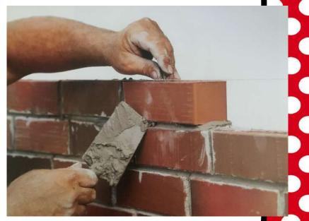
In this picture, you can see a bricklayer laying bricks the way it was done three hundred years ago. He is using a special tool called a trowel to spread the mortar. Mortar is a really gooey, sticky material made of sand, water, and a type of crushed rock called lime. Once the bricklayer has spread mortar evenly with his trowel, he will add another brick to
