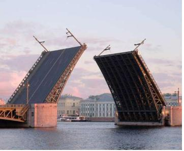
Some bridges tilt up to open on one side. Some bridges have two pieces tilt up to open in the middle.
