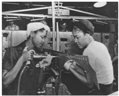
These women were working as riveters. Rivets are heavy bolts that hold pieces of metal together.
