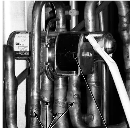
Brazed parts of 4-way valve R.V. coil
