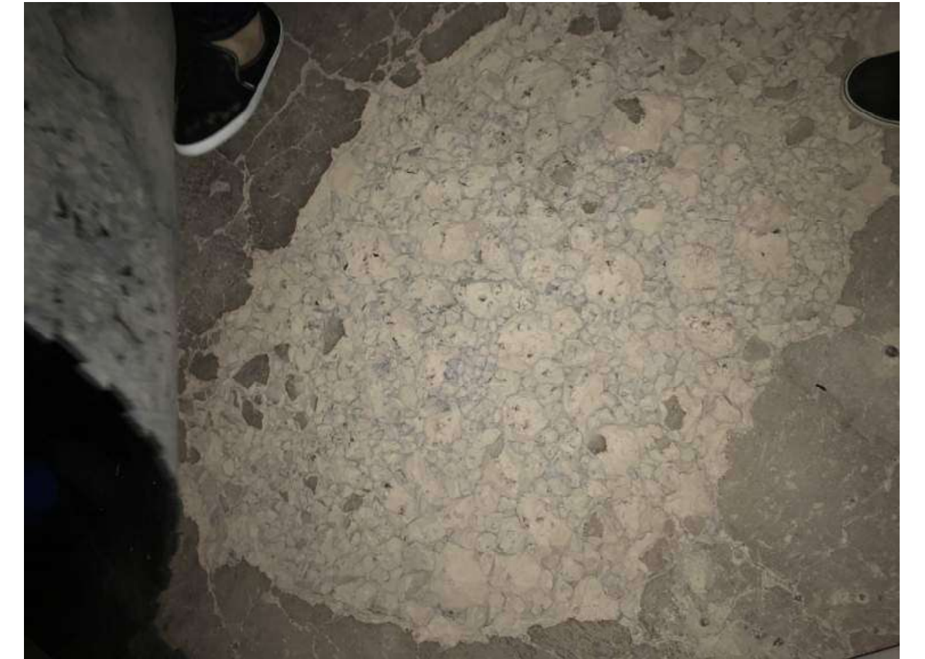
Figure 5. Deteriorated Concrete Floor Slab in Weight Room (1985 Addition)
