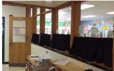
Glazing at Kindergarten
