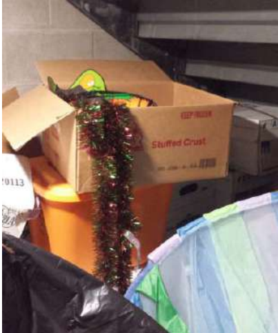
Storage under egress stairs
