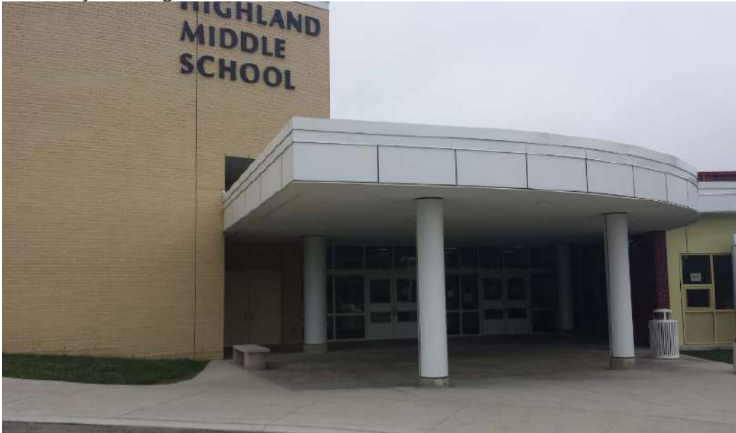
Front Façade Image
