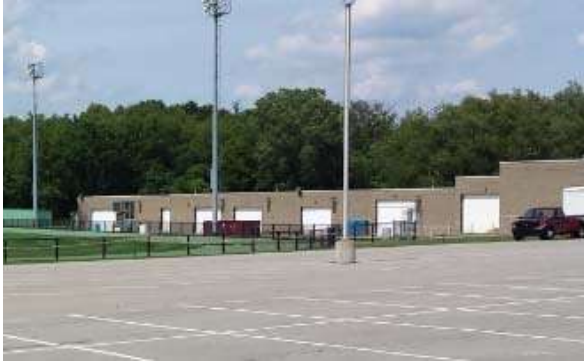
Front Façade Image
