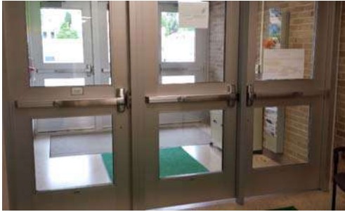
Main vestibule doors
