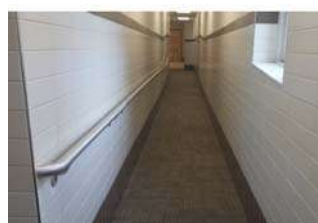
Code Compliant Ramp
