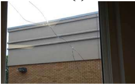
Cracked glazing
