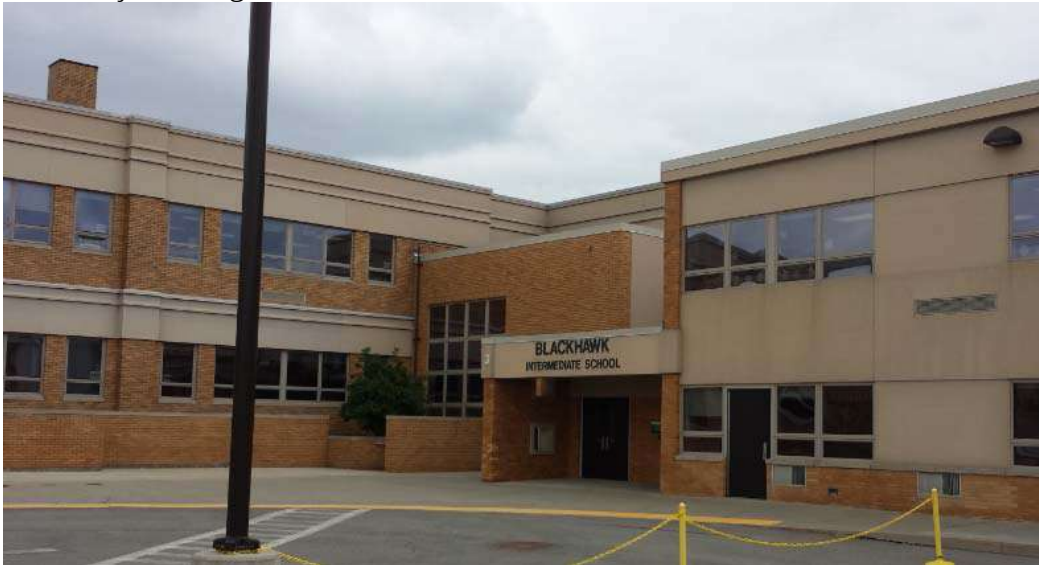
Front Façade Image
