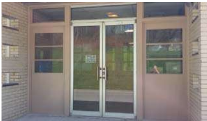
Glazing at secondary doors
