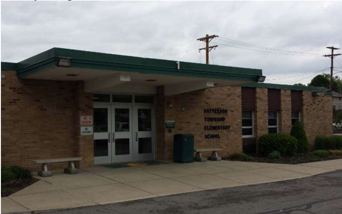
Front Façade Image
