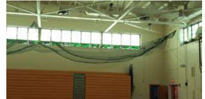
Painted gym windows
