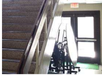
Items stored in stairs
