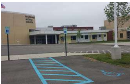
Main Entry Accessible Route
