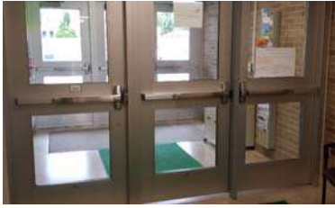
Main egress doors
