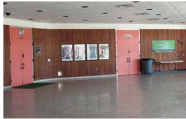
Paneling at walls
