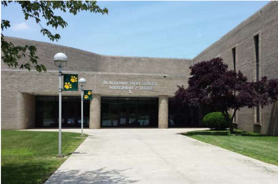
Front Façade Image
