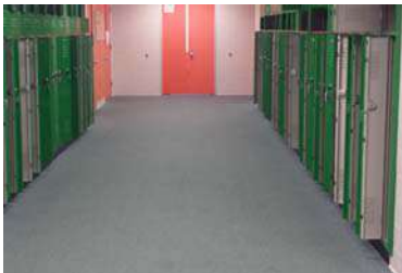
2 nd Floor corridor flooring
