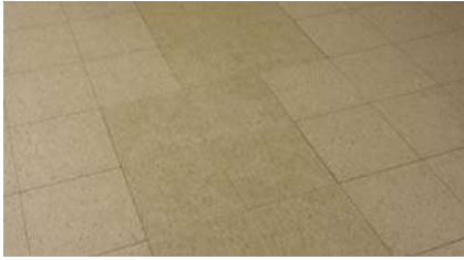
Floor tile patching
