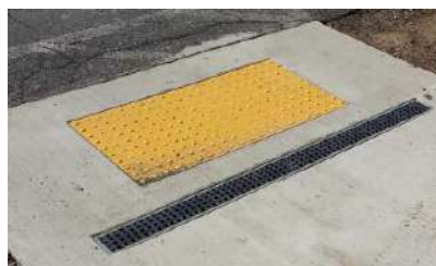
Tactile warning strips
