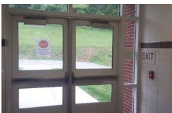
Code Compliant Exit
