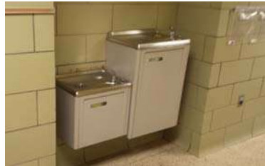
Non-compliant water cooler
