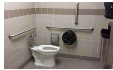
Compliant single user toilet
