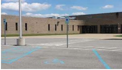
Rear entry accessible route
