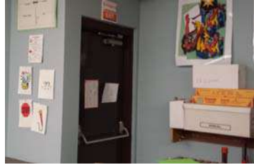
Direct exit from classroom
