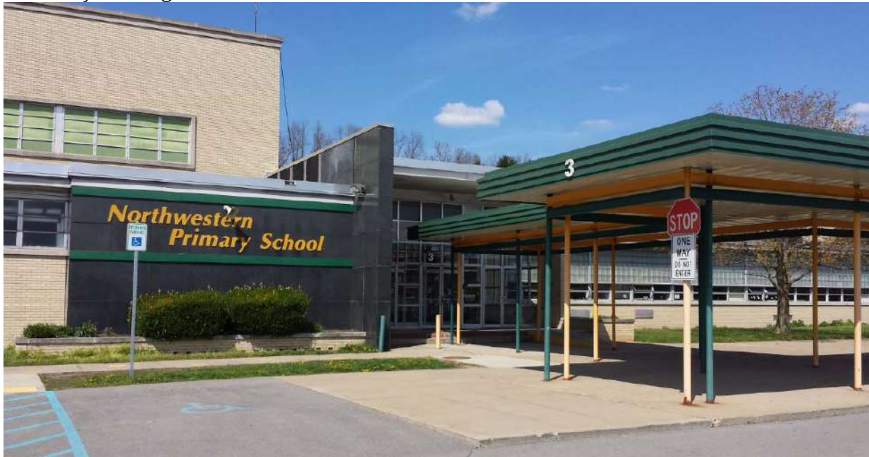
Front Façade Image
