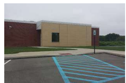
Rear Accessible Entry
