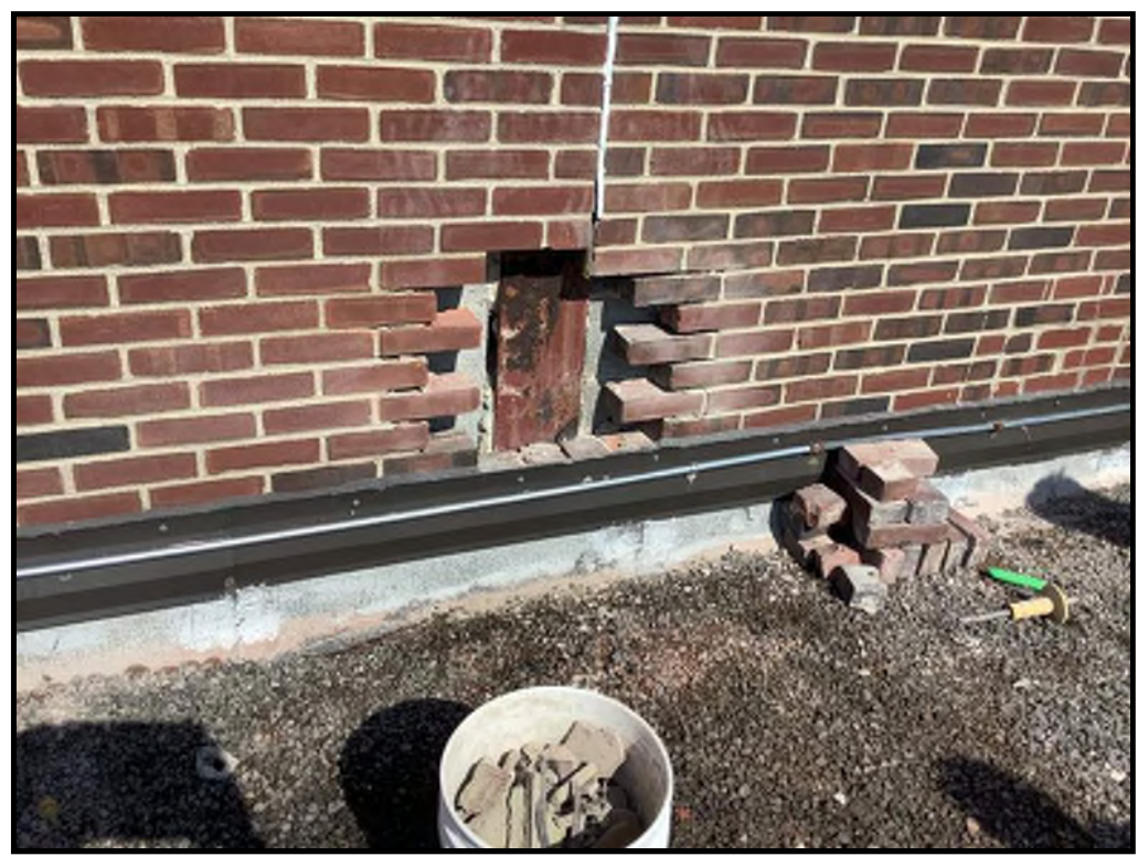
M3 ITEM 405C - FLASHING REPAIRS - SOUTH GYMNASIUM EAST ELEVATION
