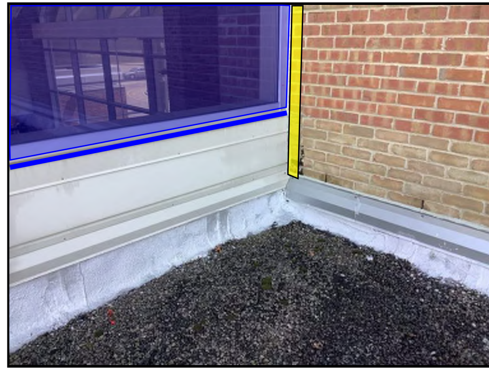
K9 ITEMS 405F, 792C, 792D - SOUTH ENTRANCE CURTAIN WALL CAVITY CLOSURE AND SEALANT REPAIR - CORNER
