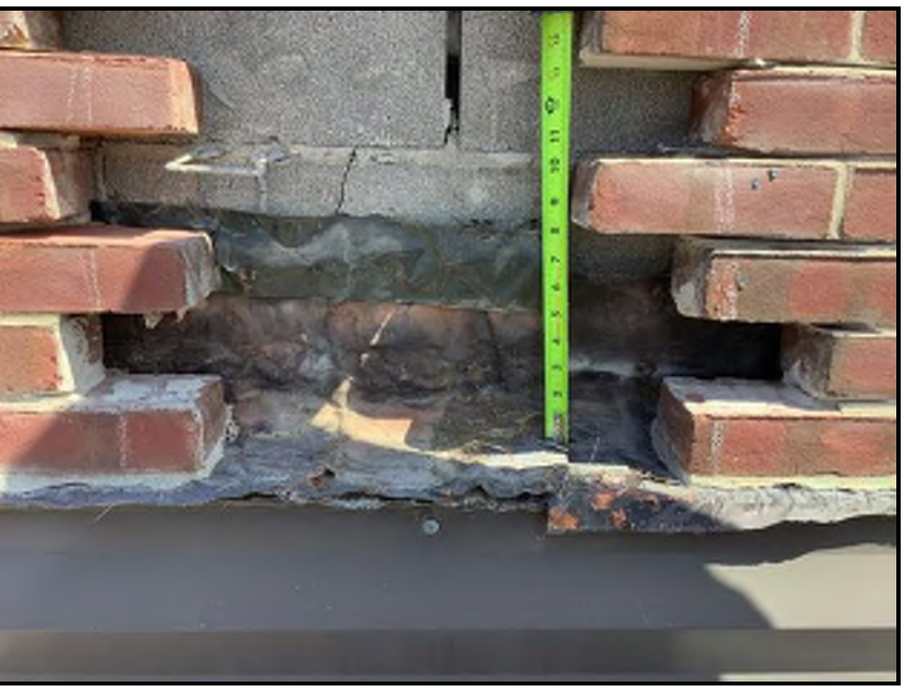
M5 ITEM 405C - FLASHING REPAIRS - NORTH GYMNASIUM SOUTH ELEVATION
