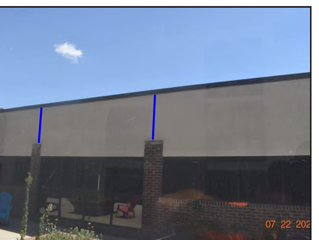
M29 792F - SEALANT REPLACEMENT AT EIFS PANEL JOINTS
