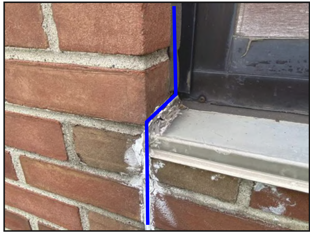
C6 ITEM 792A - SEALANT REPLACEMENT AT DISSIMILAR MATERIALS - BRICK-TO-FRAME JOINTS
