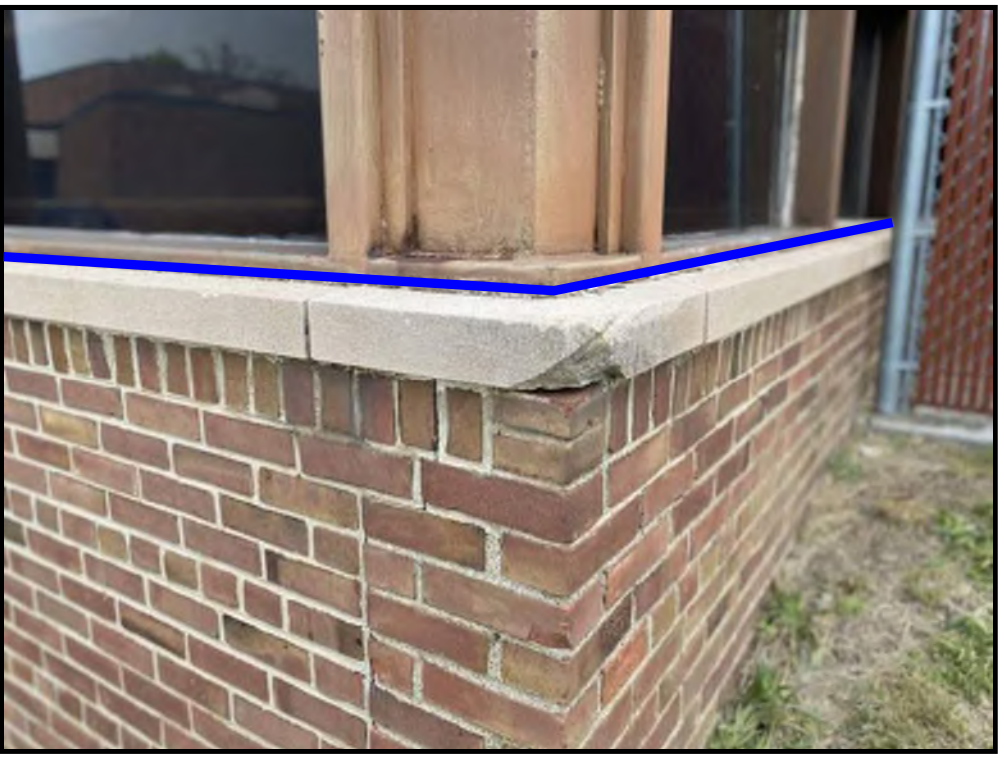
C10 ITEM 792D - SEALANT REPLACEMENT AROUND OPENINGS
