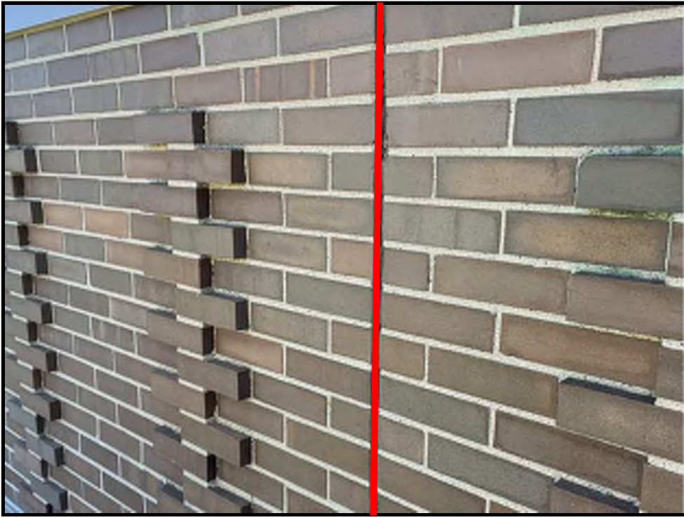
KM7 ITEM 795 - SEALANT REPLACEMENT AT TYPICAL EXPANSION JOINT
