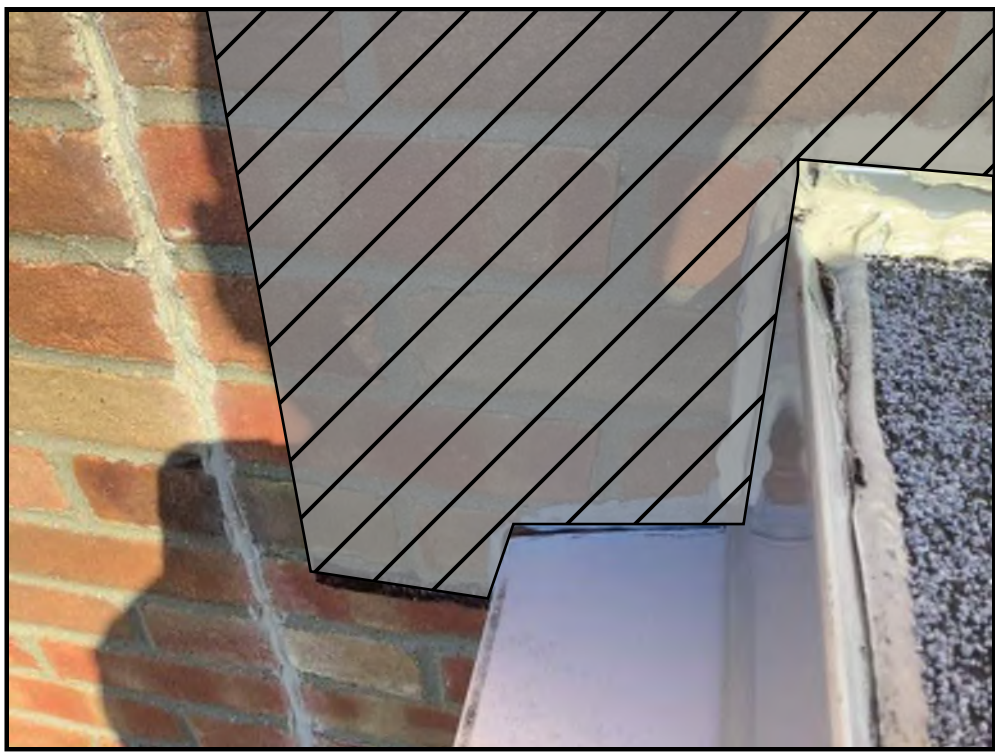
K2 ITEM 405C6 - PAC SOUTH ELEVATION FLASHING REPAIR
