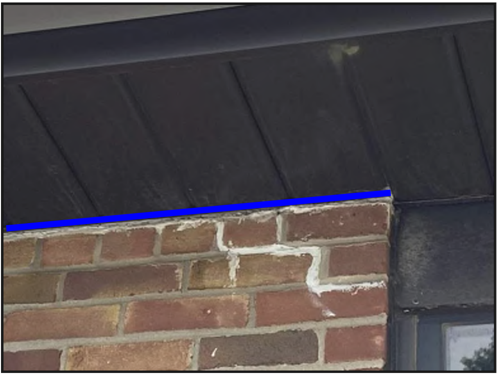
C7 ITEM 792A - SEALANT REPLACEMENT AT DISSIMILAR MATERIALS - BRICK-TO-SOFFIT JOINTS
