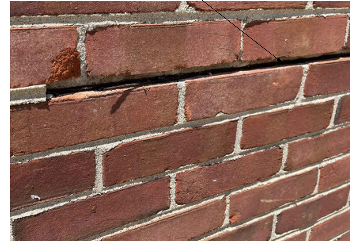
405B GRIND HORIZONTAL REINFORCING & REPOINT NOT TO SCALE
