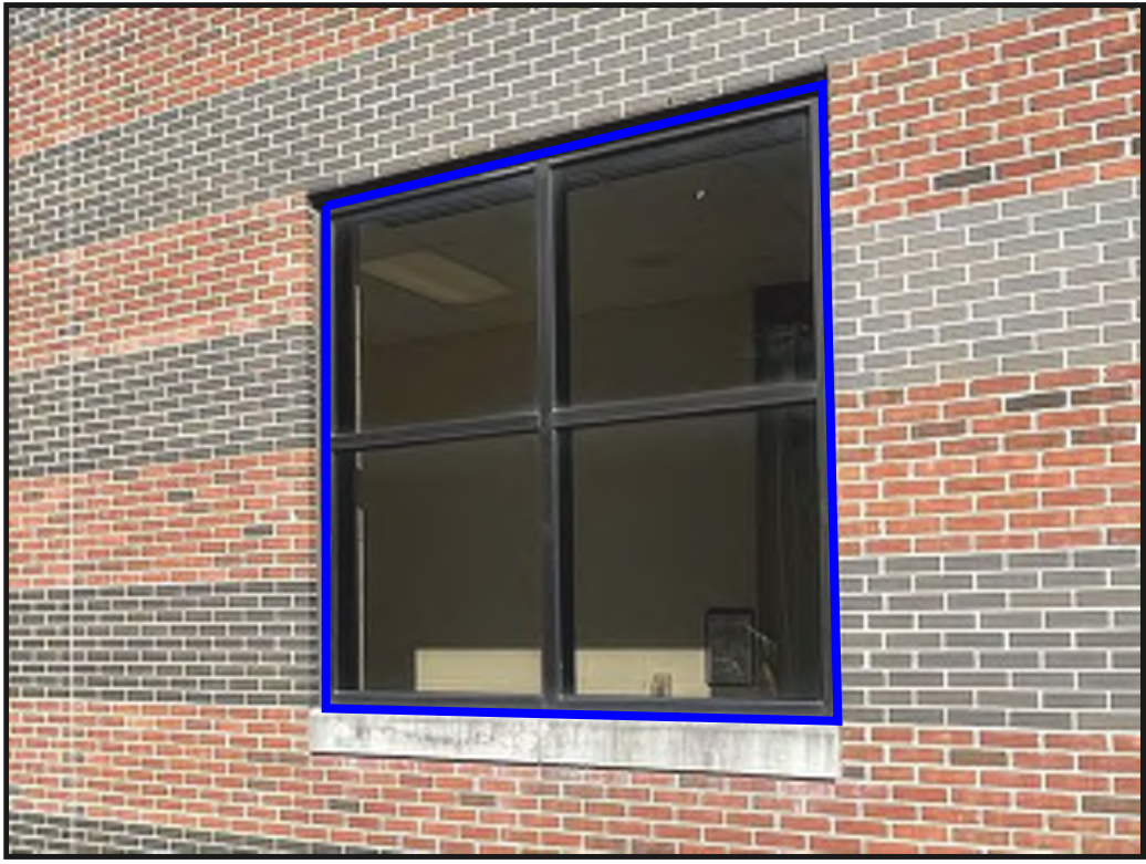
M21 ITEM 792D - SEALANT REPLACEMENT AROUND OPENINGS - WINDOWS
