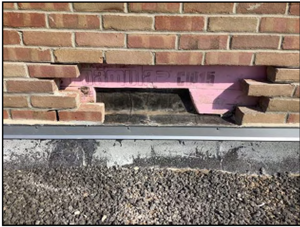
K3 ITEM 405C6 - PAC SOUTH ELEVATION FLASHING REPAIR EXISTING CONDITIONS NO. 3
