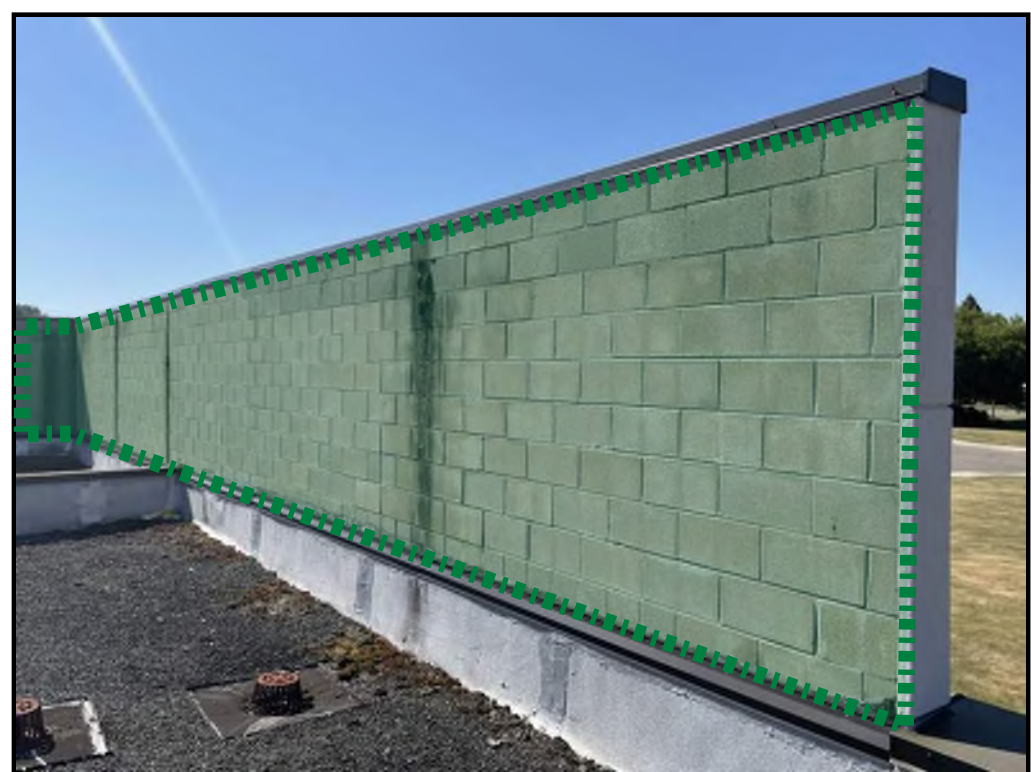
M9 ITEM 996 - CMU ELASTOMERIC COATING REPAIRS
