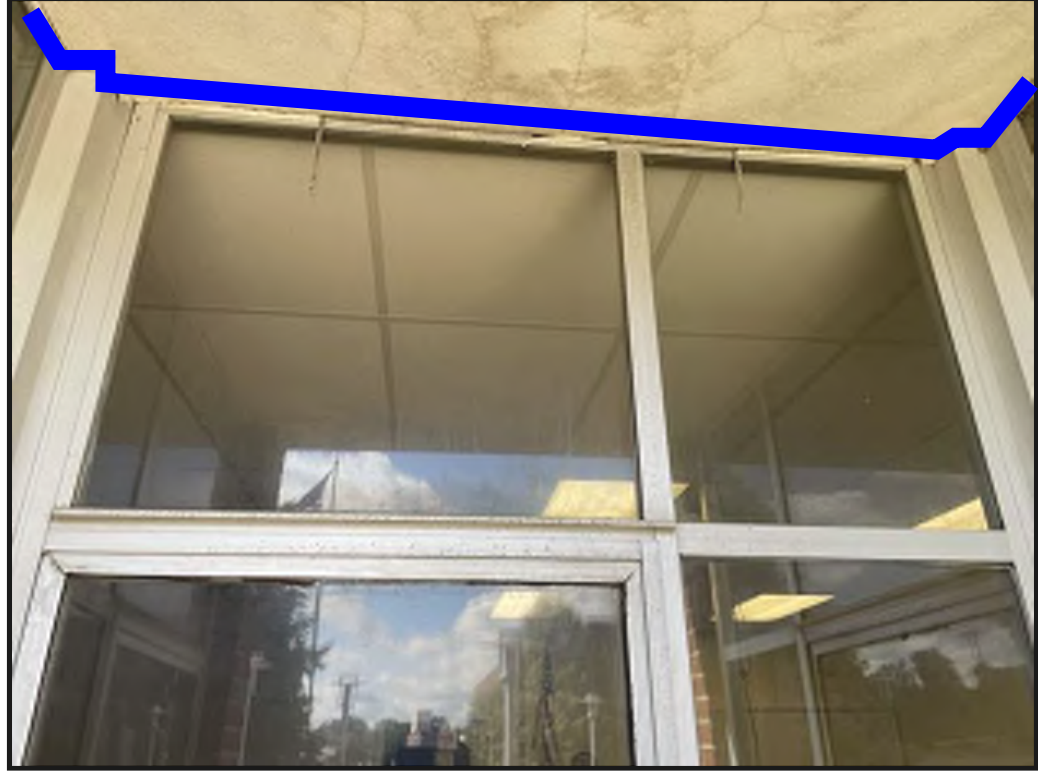
M24 ITEM 792A - SEALANT REPLACEMENT AT DISSIMILAR MATERIALS - FIBERBOARD-TO-FRAME JOINTS
