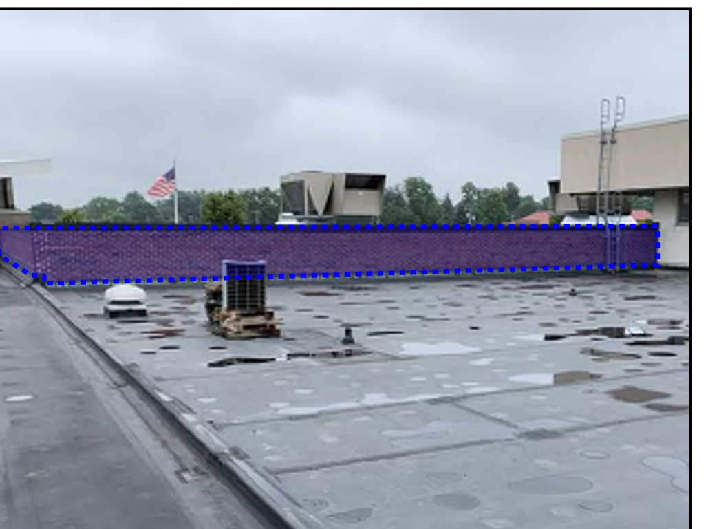
M13 ITEM 405A - BRICK REPOINTING AT PARAPET
