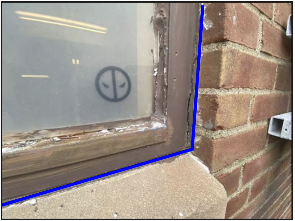
C11 ITEM 792D - SEALANT REPLACEMENT AROUND OPENINGS
