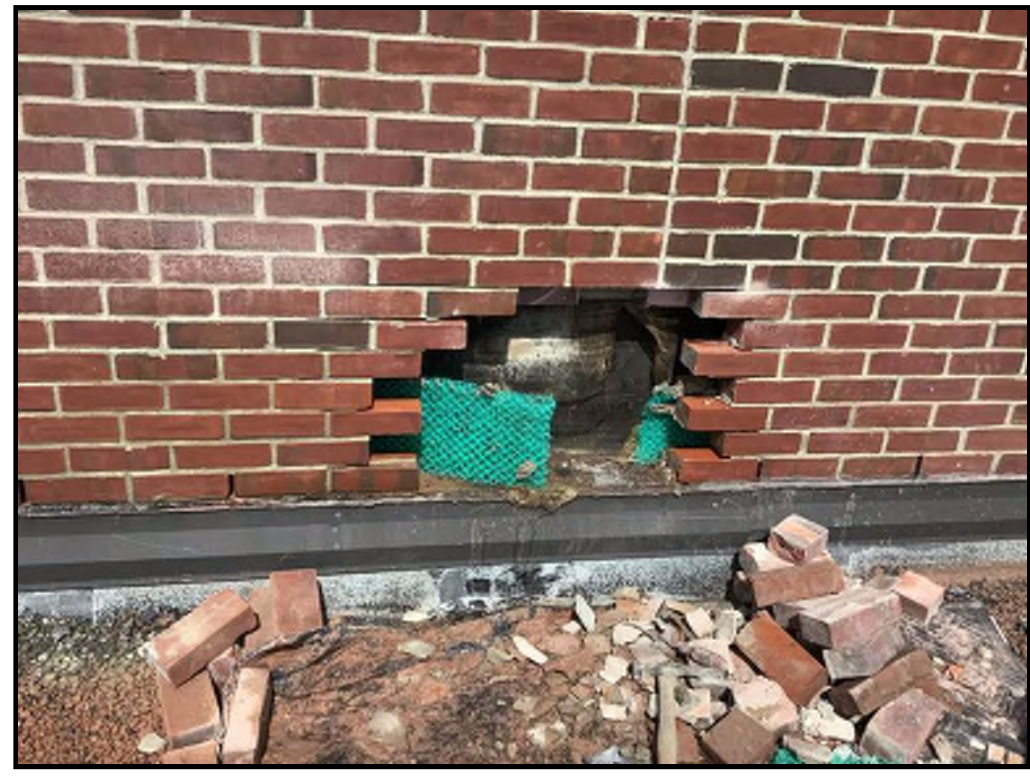
M1 ITEM 405C - FLASHING REPAIRS - PERFORMING ARTS CENTER
