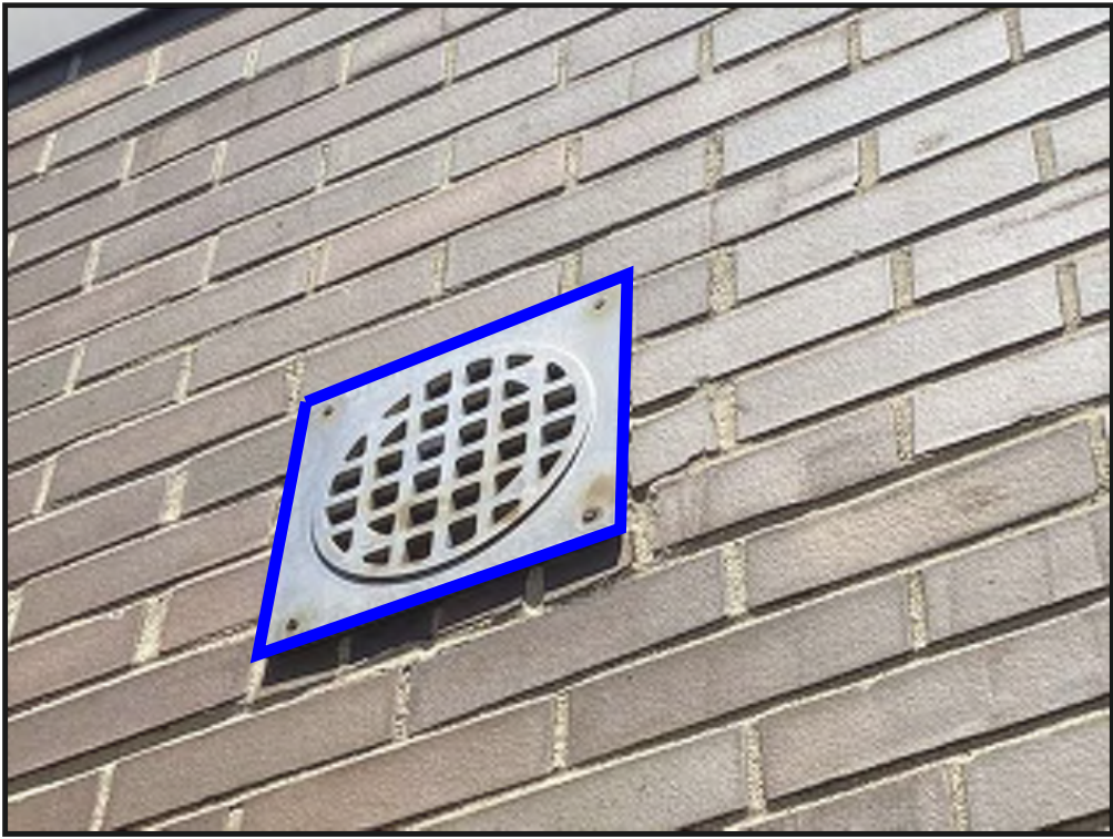
KM2 ITEM 792D - SEALANT REPLACEMENT AT UNSEALED PENETRATIONS
