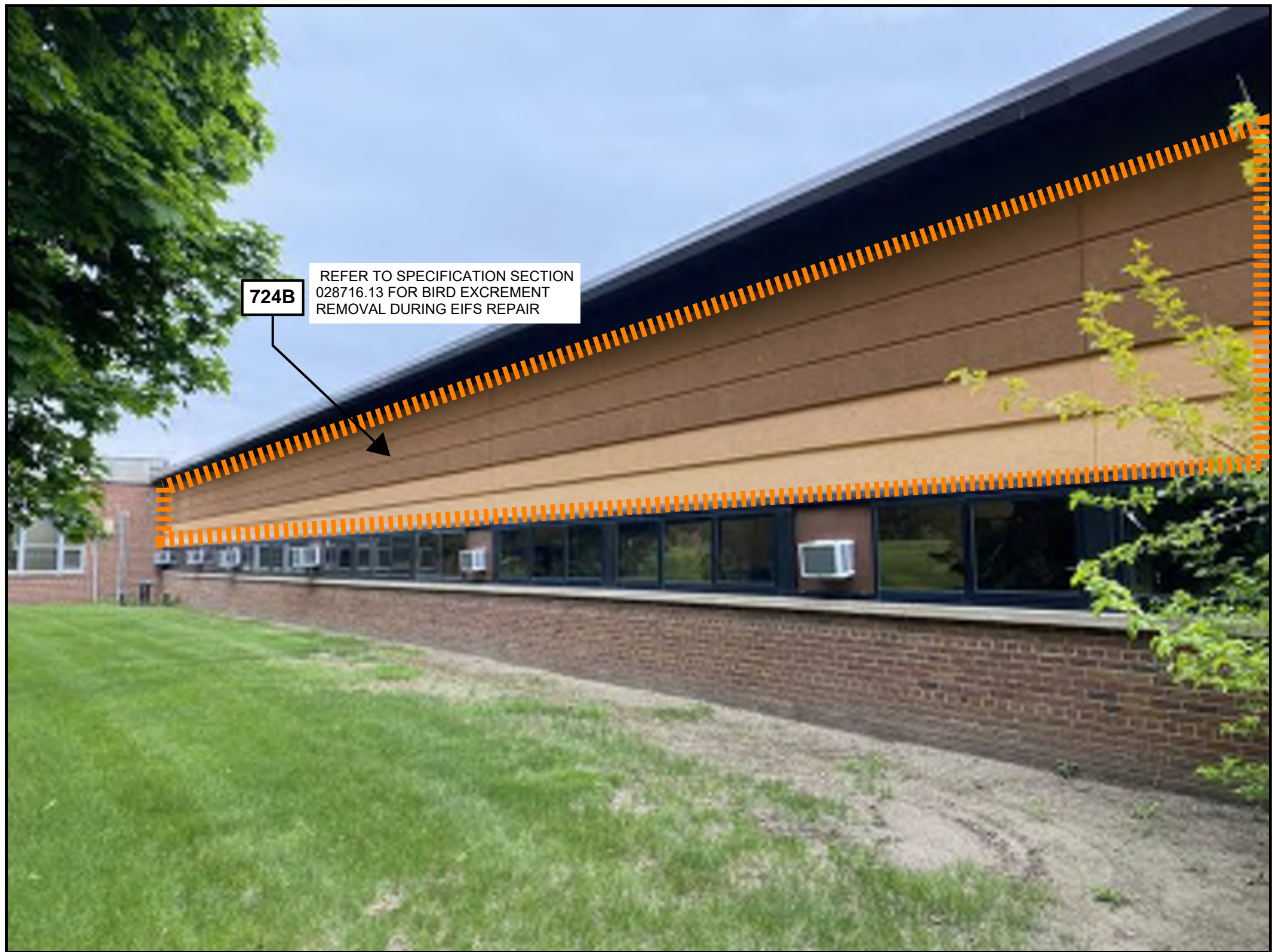
PARTIAL EAST ELEVATION EIFS REPLACEMENT
