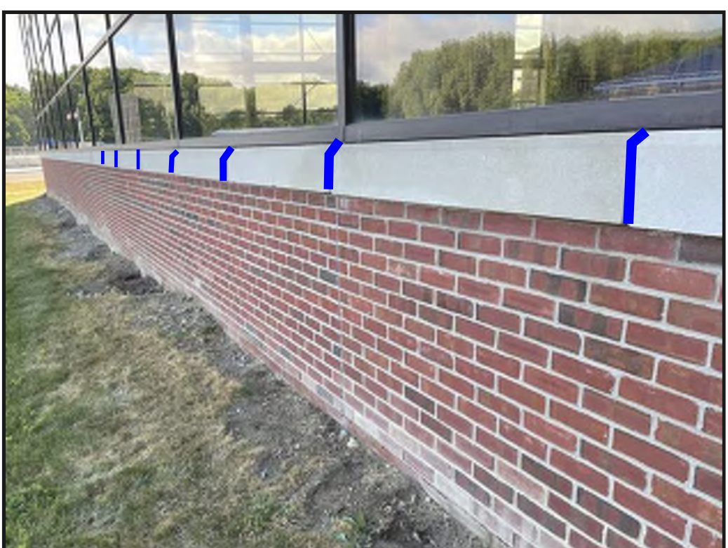
M27 ITEM 792B - SEALANT REPLACEMENT AT PRECAST WINDOWSILL JOINTS
