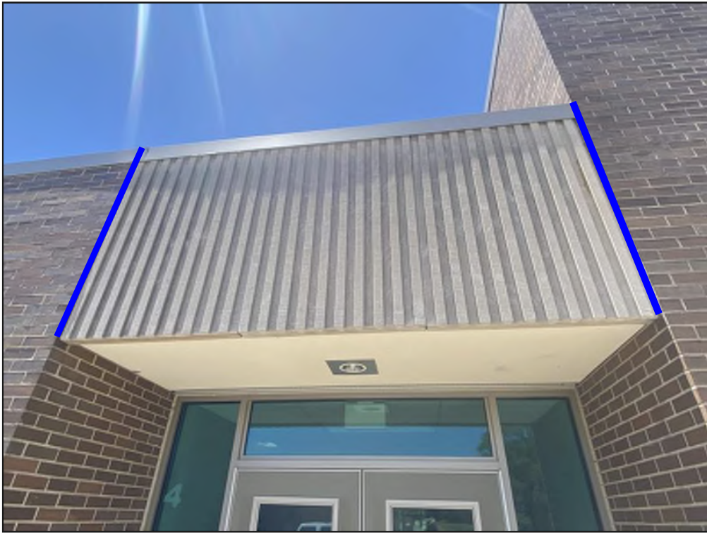
KM5 ITEM 792E - SEALANT REPLACEMENT AT DISSIMILAR MATERIALS - PRECAST PANEL JOINTS
