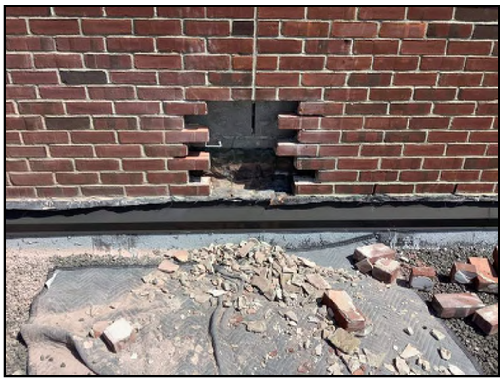
M4 ITEM 405C - FLASHING REPAIRS - NORTH GYMNASIUM SOUTH ELEVATION
