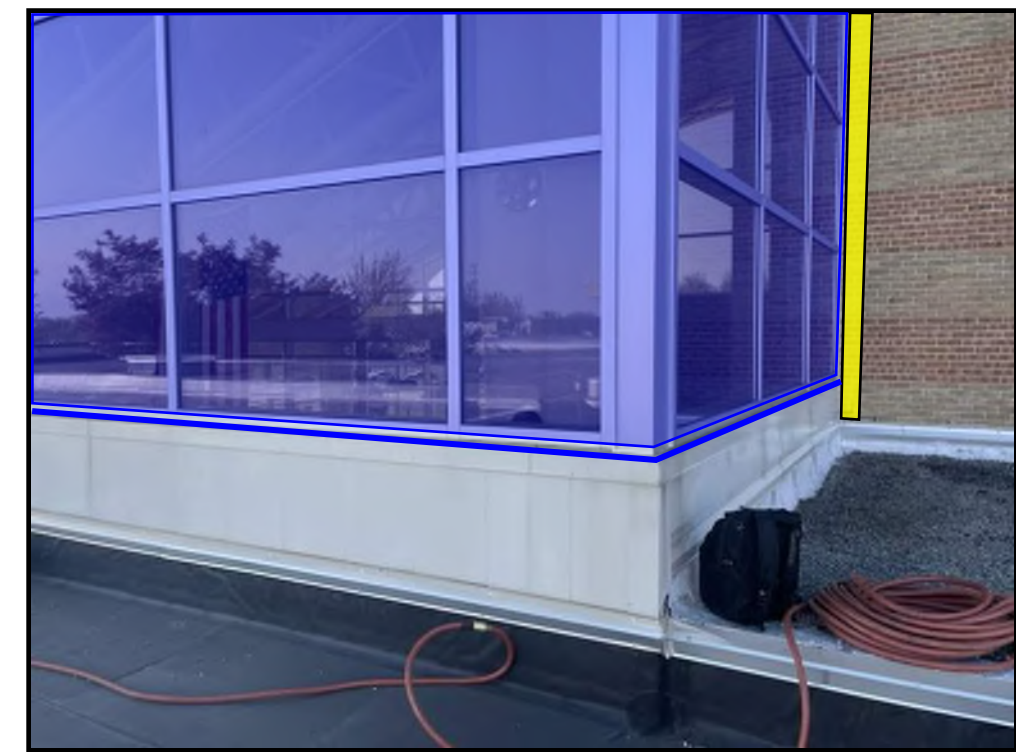
K8 ITEMS 405F, 792C, 792D - SOUTH ENTRANCE CURTAIN WALL CAVITY CLOSURE AND SEALANT REPAIR
