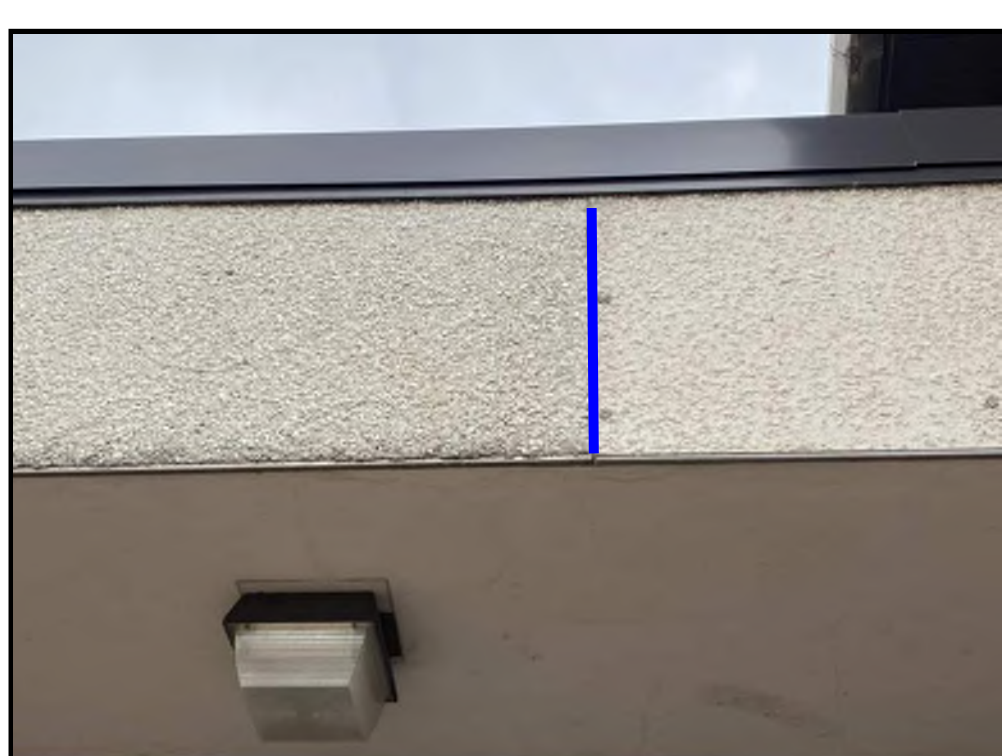
C14 ITEM 792E - PRECAST PANEL SEALANT REPLACEMENT
