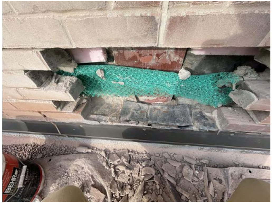
M6 ITEM 405C - FLASHING REPAIRS - NORTH GYMNASIUM EAST ELEVATION
