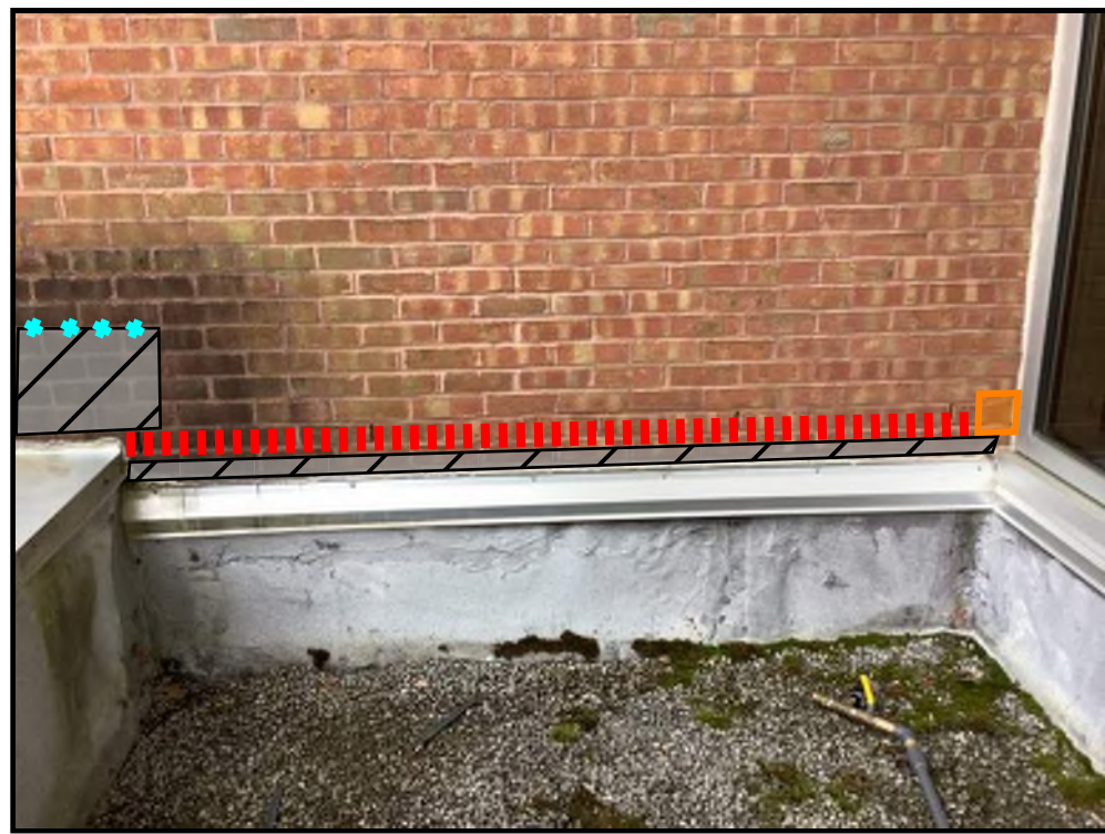
K4 ITEMS 405C, 405C4, 405E- NATATORIUM - FLASHING AND END DAM REPAIR
