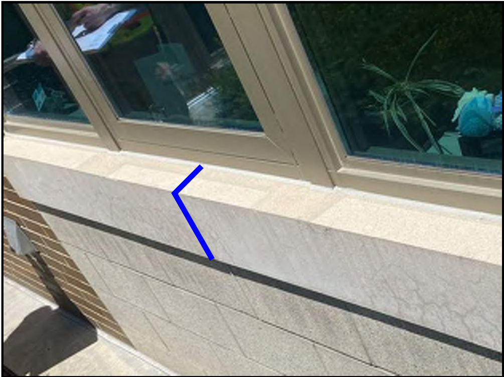
KM6 ITEM 792B - SEALANT REPLACEMENT AT PRECAST SILL
