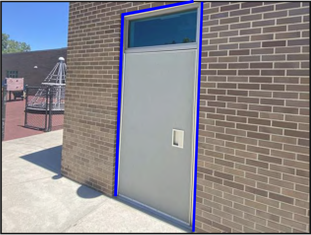
KM3 ITEM 792D - SEALANT REPLACEMENT AT DOOR PERIMETER
