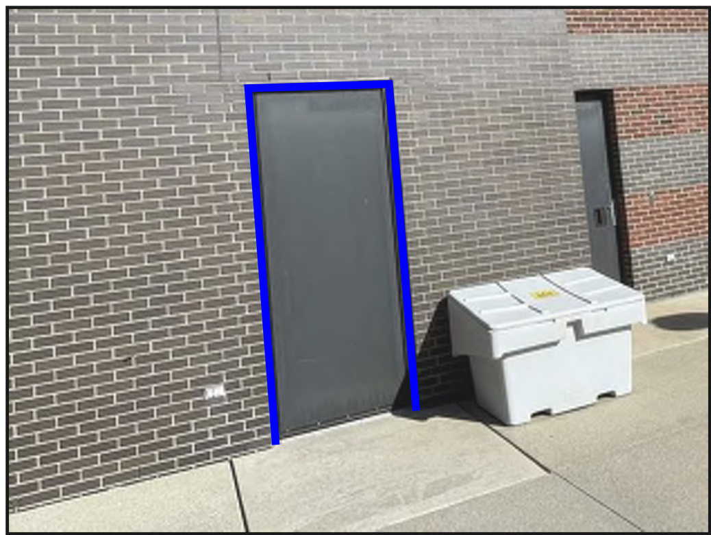
M22 ITEM 792D - SEALANT REPLACEMENT AROUND OPENINGS - DOORS
