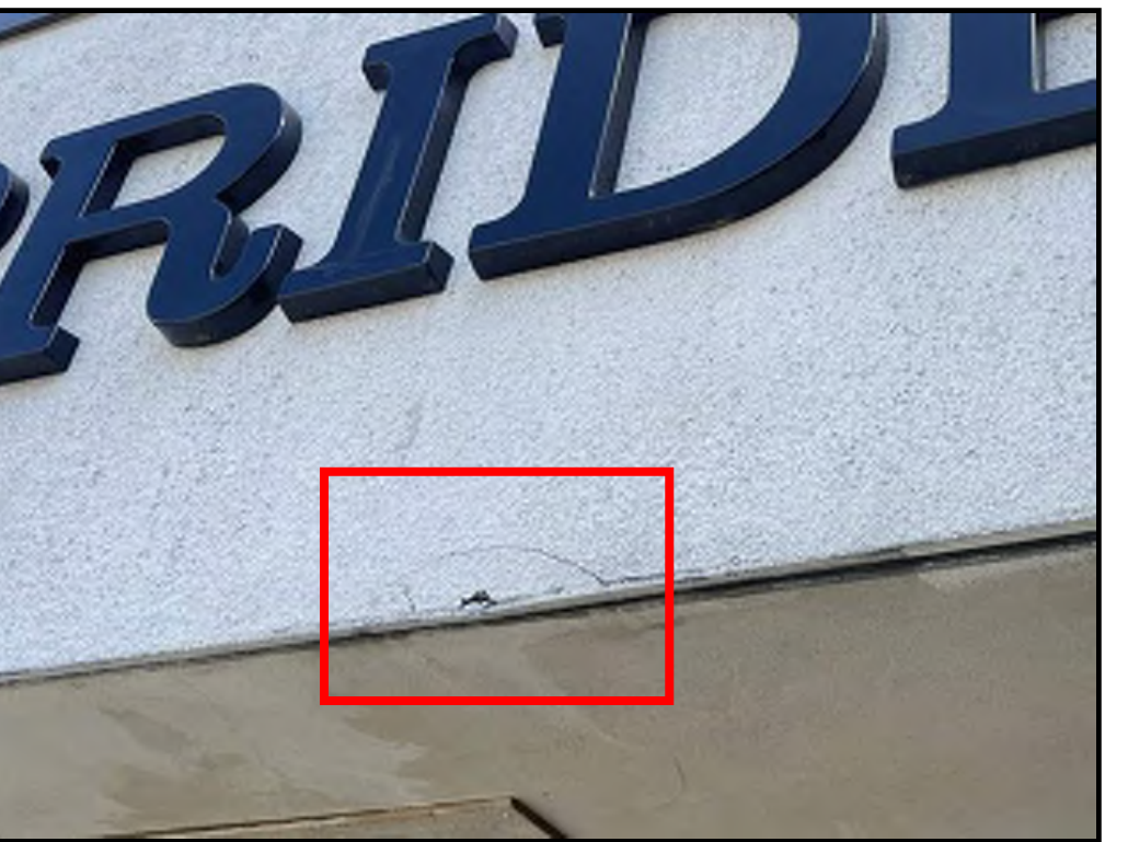
M10 ITEM 724A - CANOPY PATCH REPAIRS
