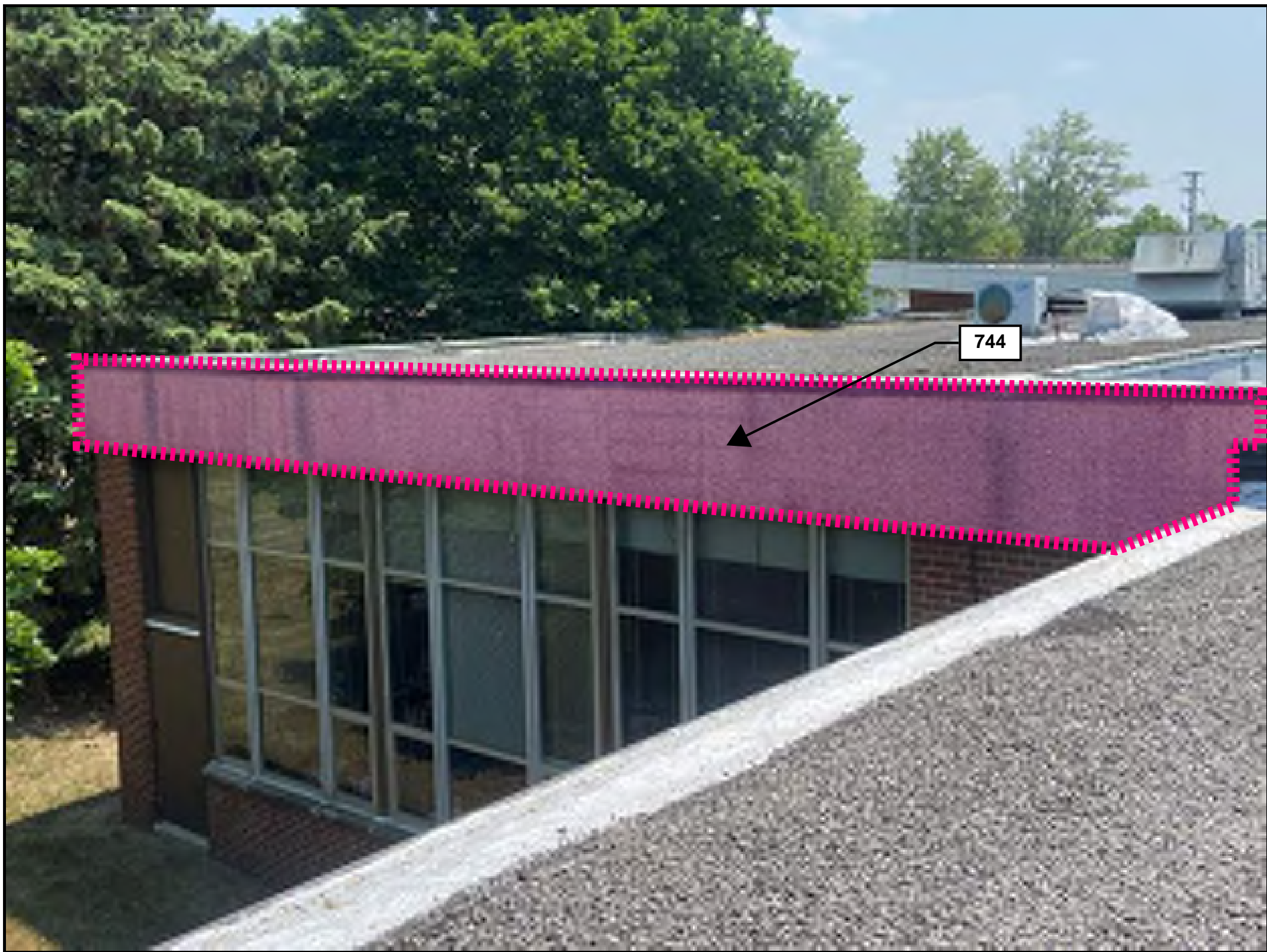
PARTIAL NORTH ELEVATION AGGREGATE COATING REPAIR
