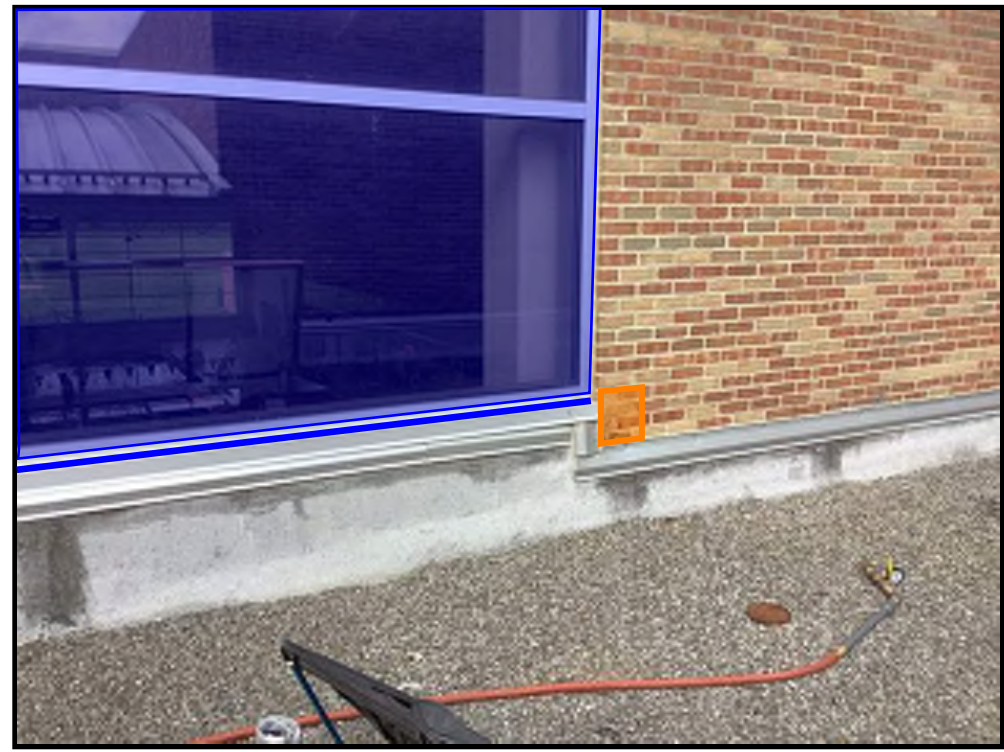
K6 ITEMS 405E, 792C, 792D - NATATORIUM SEALANT AND END DAM REPAIR - NORTH
