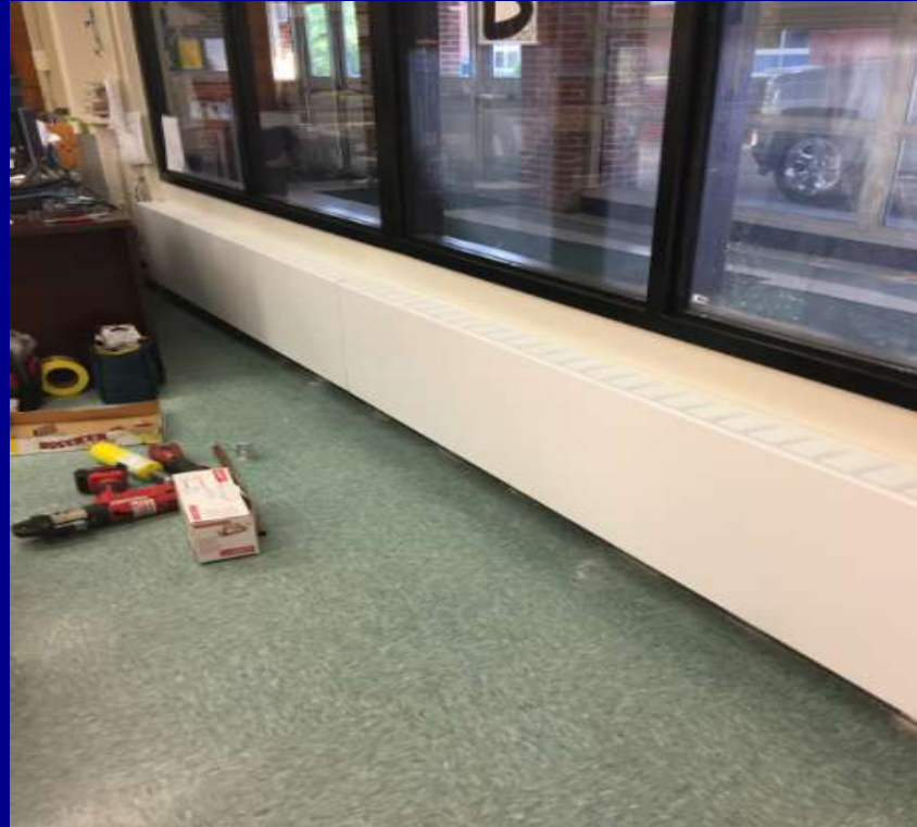
New main office radiator and cover installation along new window elevation
