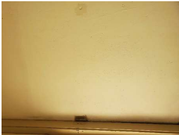
Photo #5 HA# D 10 – Acoustical Plaster Ceilings
