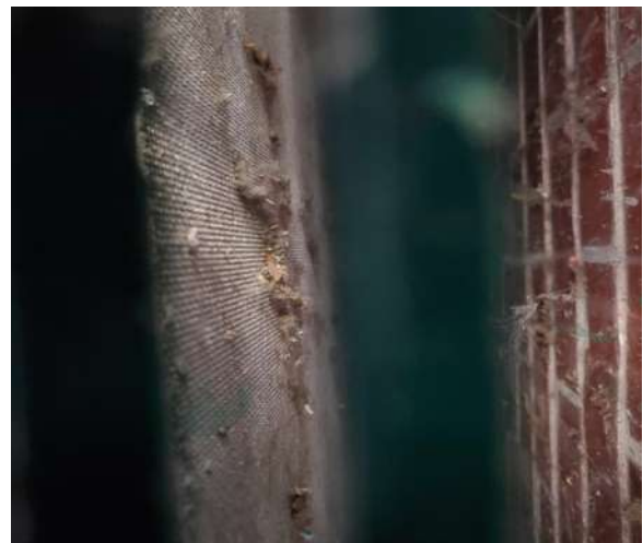
Photo #6 HA# C 10 – Heating Cabinet Liner Panels
