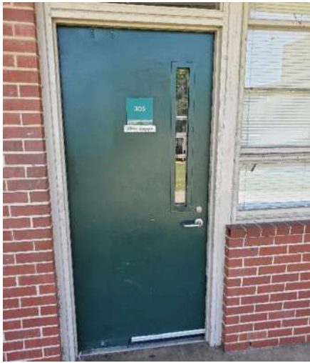
Photo #7 HA# C 11 – Fire Doors (multiple types)
