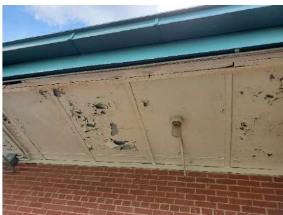
Photo #5 HA# F 13 – Cementitious Panels
