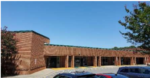
Photo #1 Building I Exterior
