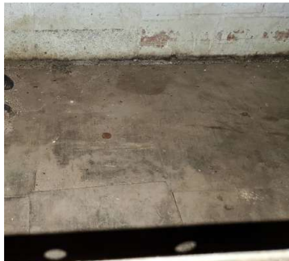
Photo #6 HA# G 8 – 9"x9" Floor Tile and Mastic (Old Gym)
