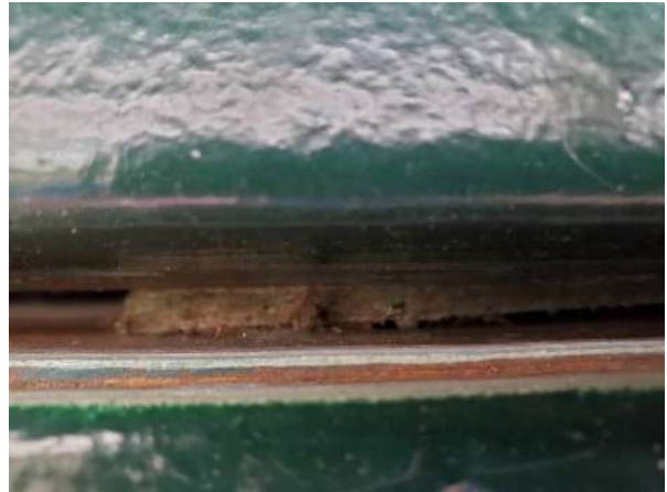
Photo #6 HA# D 11 – Heating Cabinet Liner Panels
