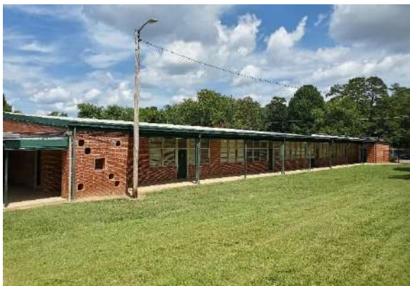
Photo #1 Building D Exterior
