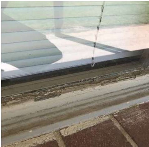
Photo #3 HA# C 7 – Exterior Window Glazing
