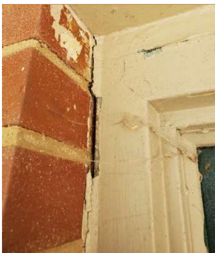
Photo #3 HA# H 8 – Exterior Door Caulk
