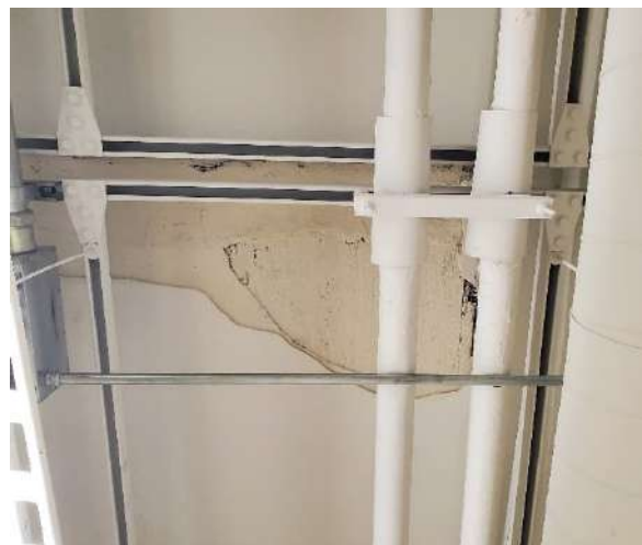
Photo #6 HA# A 24 – Acoustical Plaster Ceilings
