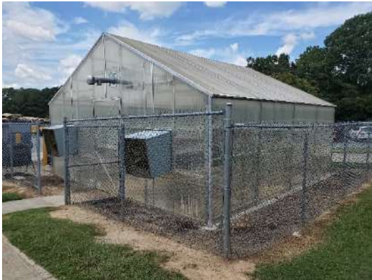
Photo #1 Greenhouse Exterior
