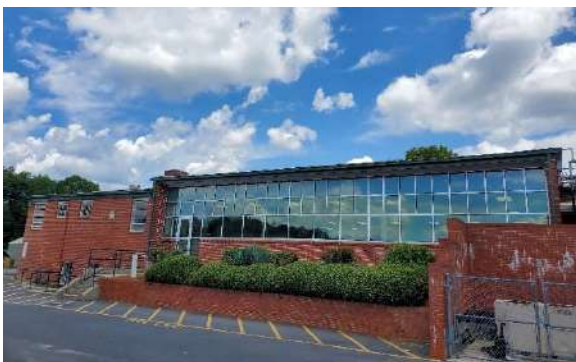
Photo #1 Building E Exterior
