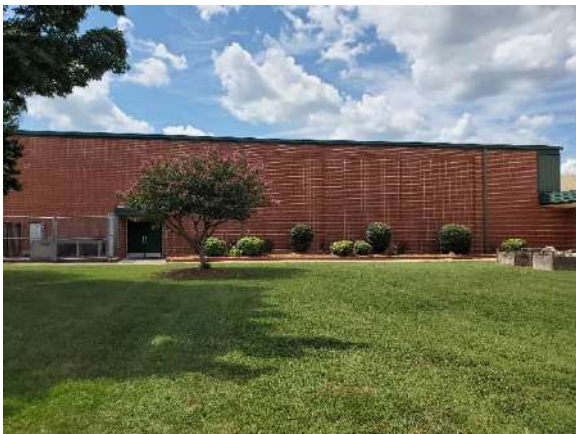
Photo #1 Building B Exterior
