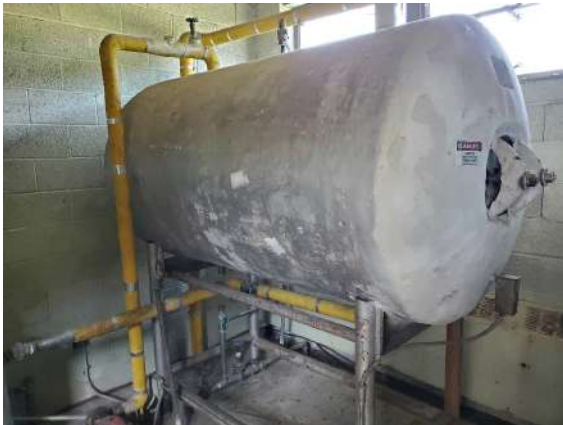
Photo #7 HA# G 9 – Tank Insulation (Old Gym)
