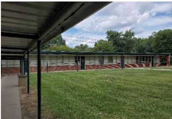
Photo #1 Building H Exterior
