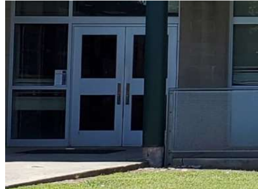
Photo #2 HA# MC 12 – Fire Doors (multiple types)
