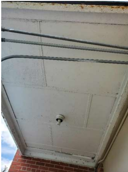
Photo #9 # A 27 – Cementitious Panels
