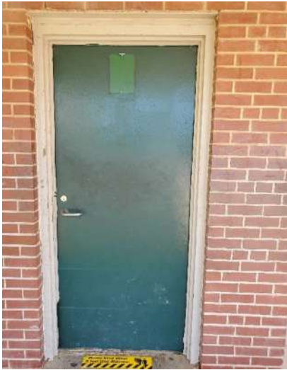
Photo #5 HA# H 10 – Fire Doors (multiple types)
