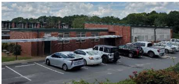
Photo #1 Building F Exterior
