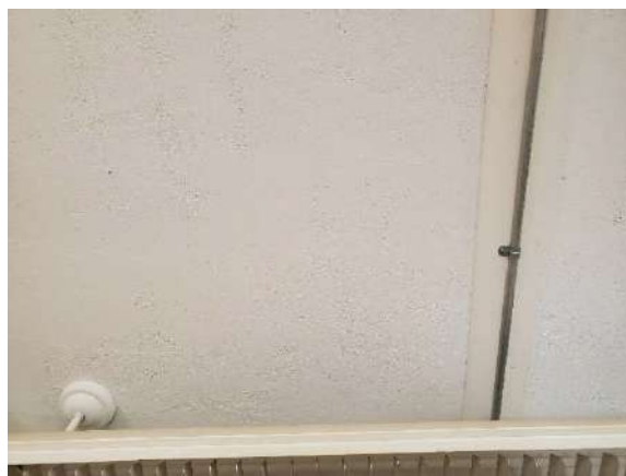
Photo #4 HA# F 12 – Acoustical Plaster Ceilings
