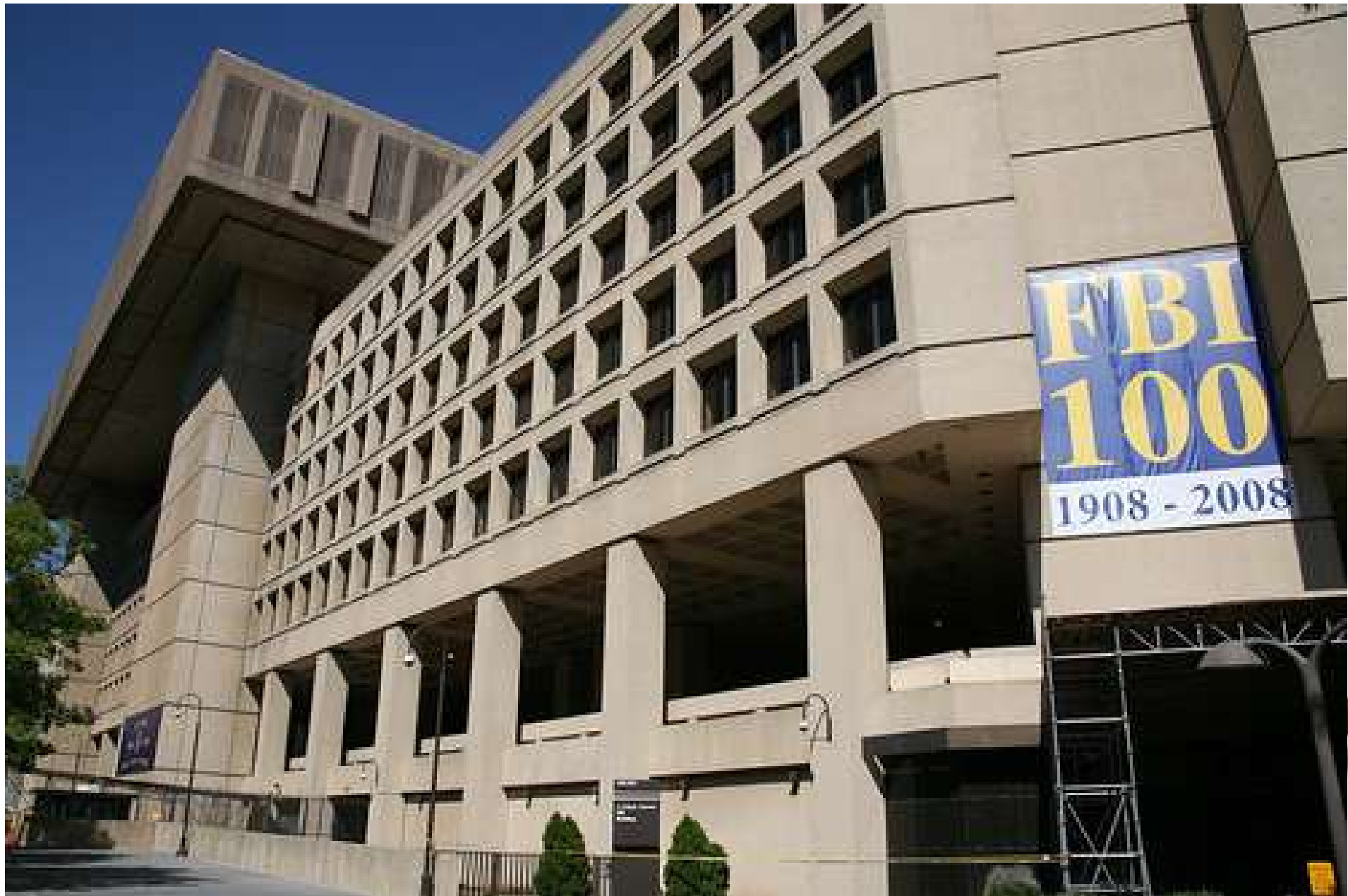
FBI Building Washington, DC
